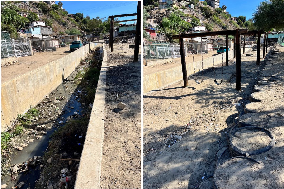
Figure 1-10 and 1-11 transit stop and local park next to the channel (32.511724,-117.086461)
