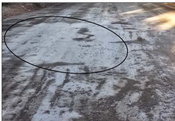
Figure 3.8: CR32B: Wet section after repair.
