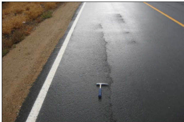
Figure 2.2: Longitudinal crack.
