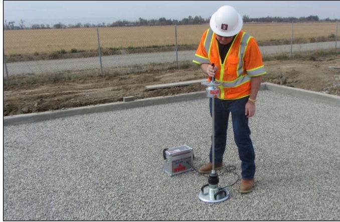
Figure 2.12: Light weight deflectometer.
