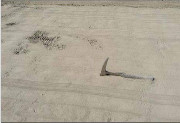
Figure 3.20: PLU147: Depth of 4% cement after spreading ( \pm 50 mm).
