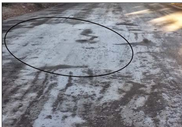
Figure 3.8: CR32B: Wet section after repair.
