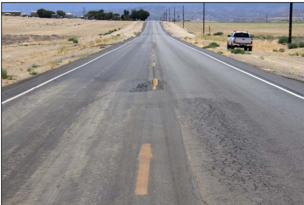
Figure 2.5: Fatigue cracking.
