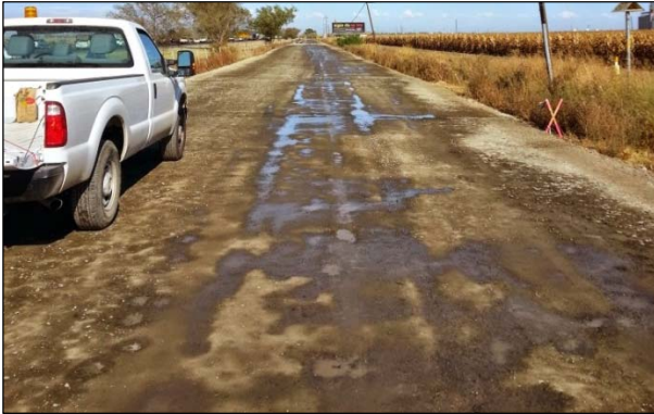
Figure 3.5: CR32B: Surface raveling.
