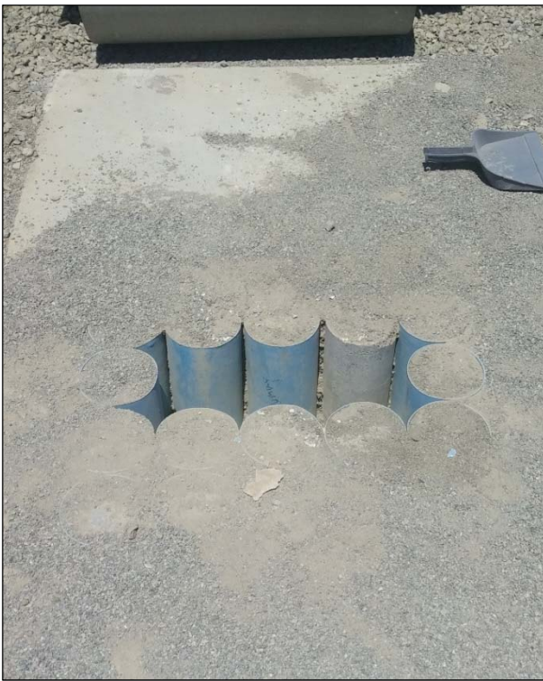
Figure 5.5: Test pit preparation.
