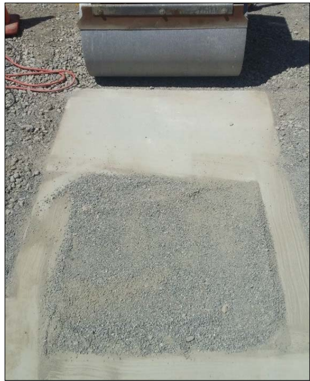
Figure 5.6: Final setup before microcracking.
