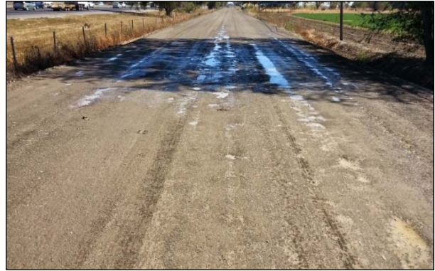
Figure 3.5: CR32B: Surface raveling.
