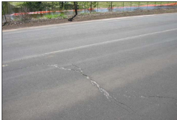
Figure 2.1: Transverse crack.
