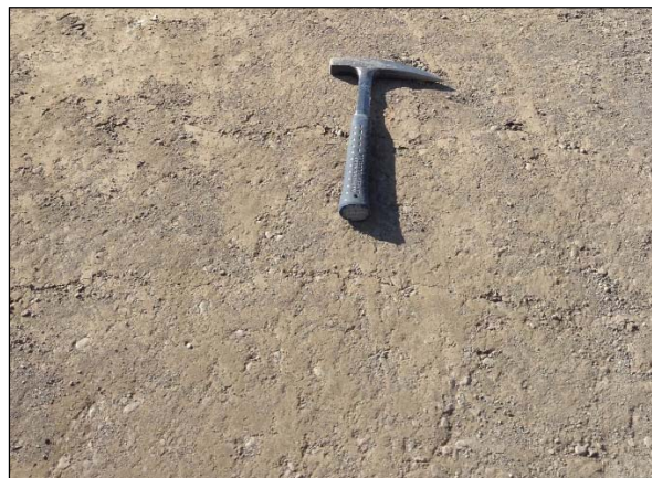
Figure 3.15: CR99: Block cracking after microcracking.
