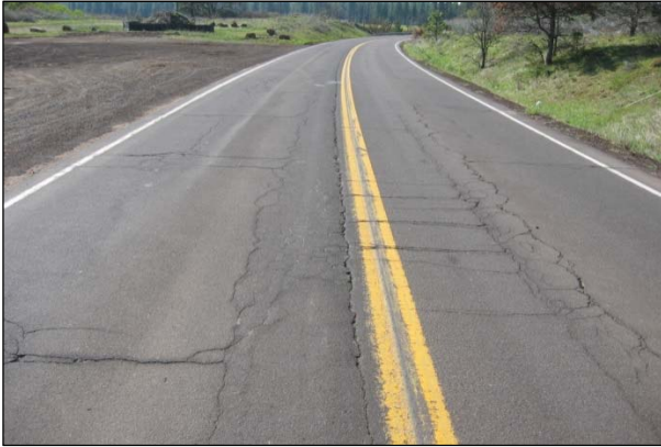
Figure 2.3: Block cracking.
