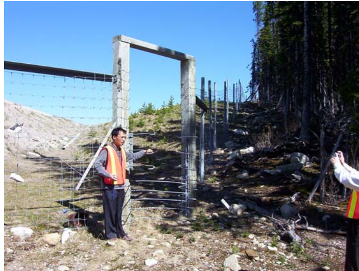
Figure 4. One-way gate designed for moose and deer
