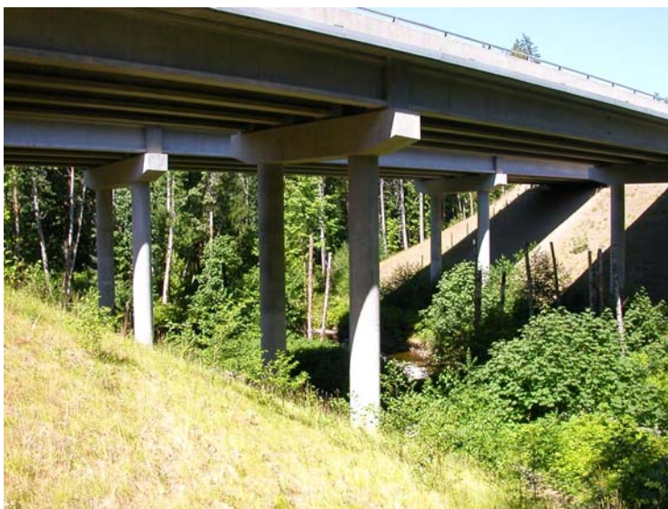
Figure 10. Multi-species wildlife underpass on the Vancouver Island Highway (1999)
