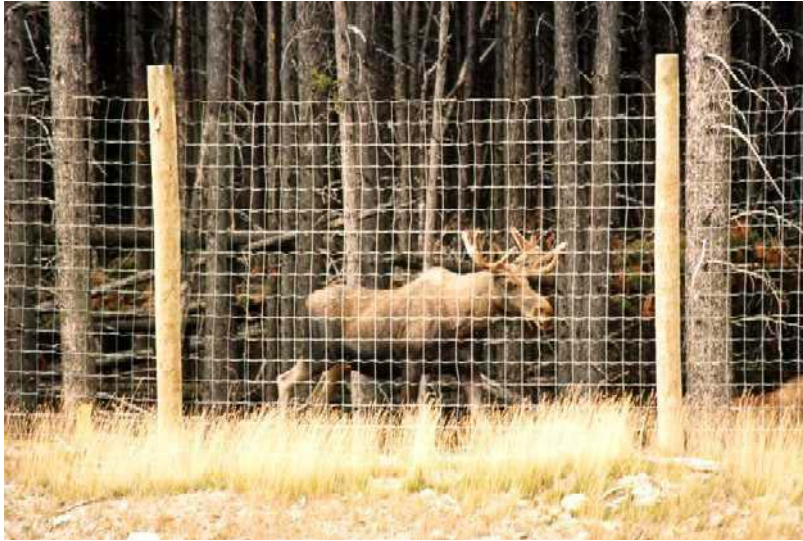
Figure 16. Wildlife exclusion fencing designed for moose
