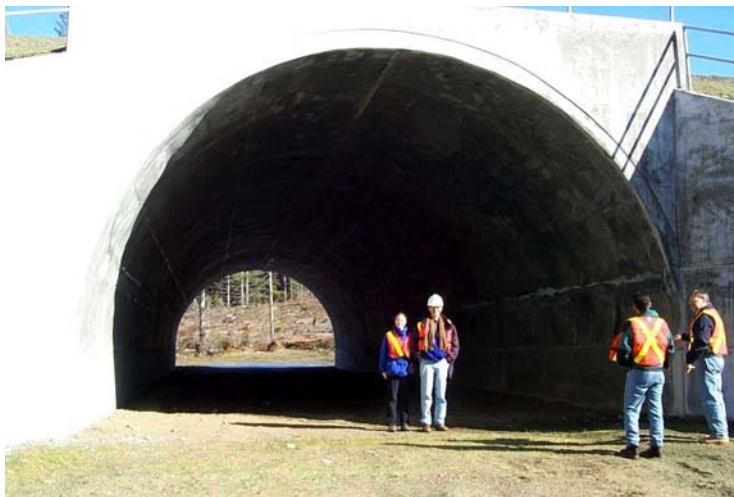
Figure 9. Wildlife underpass designed for elk and deer on the Vancouver Island Highway (1999)
