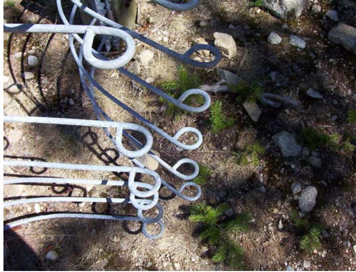
Figure 6. One-way gate with “looped” tynes
