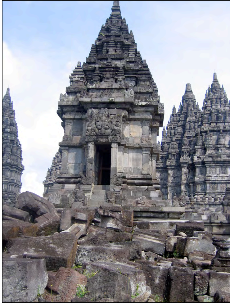
Fig. 51. The same candi from a distance. Loro Jonggrang , 2006. These pictures were taken a few days before the major 2006 earthquake that destroyed parts of the complex.
