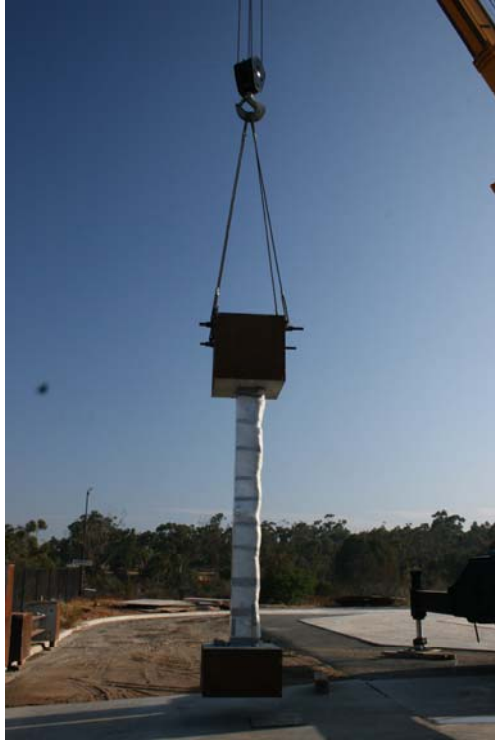
Figure 5.20: Column Craned in Place
