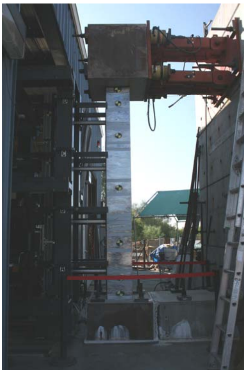
Figure 5.44: Test WA04 Column Pre-Test
