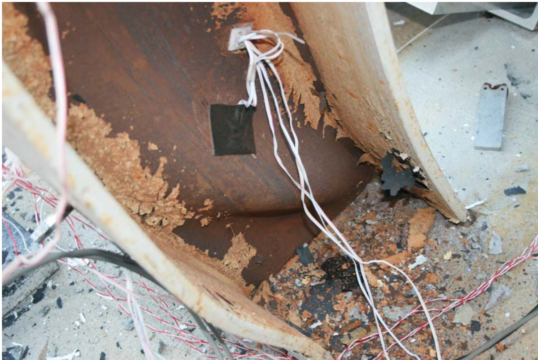
Figure 3.68: Test SA11 Column Base Post-Test (View 2)
