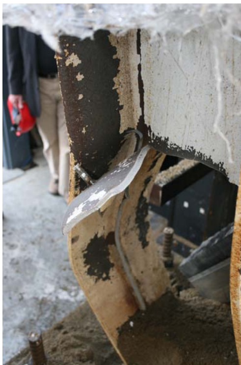
Figure 5.67: Test WA06 Column Web Fracture
