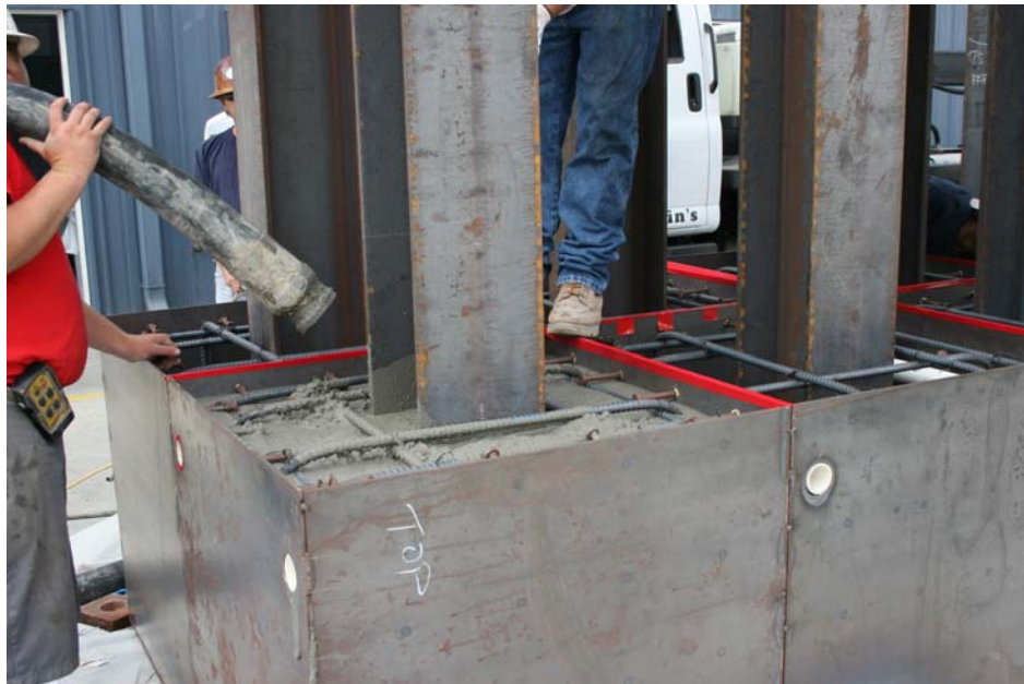
Figure 3.15: Concrete Poured into Column Header
