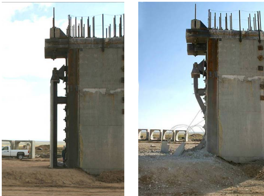
Figure 5.69: Field Test 8 Pre and Post-Test Global Deformation
