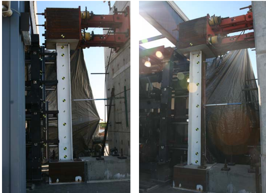
Figure 3.51: Test SA09 Column Pre-Test
