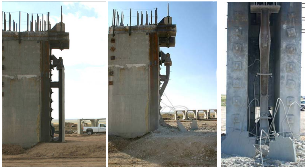
Figure 2.18: Before and After Photos from Test 9 with Cladding
