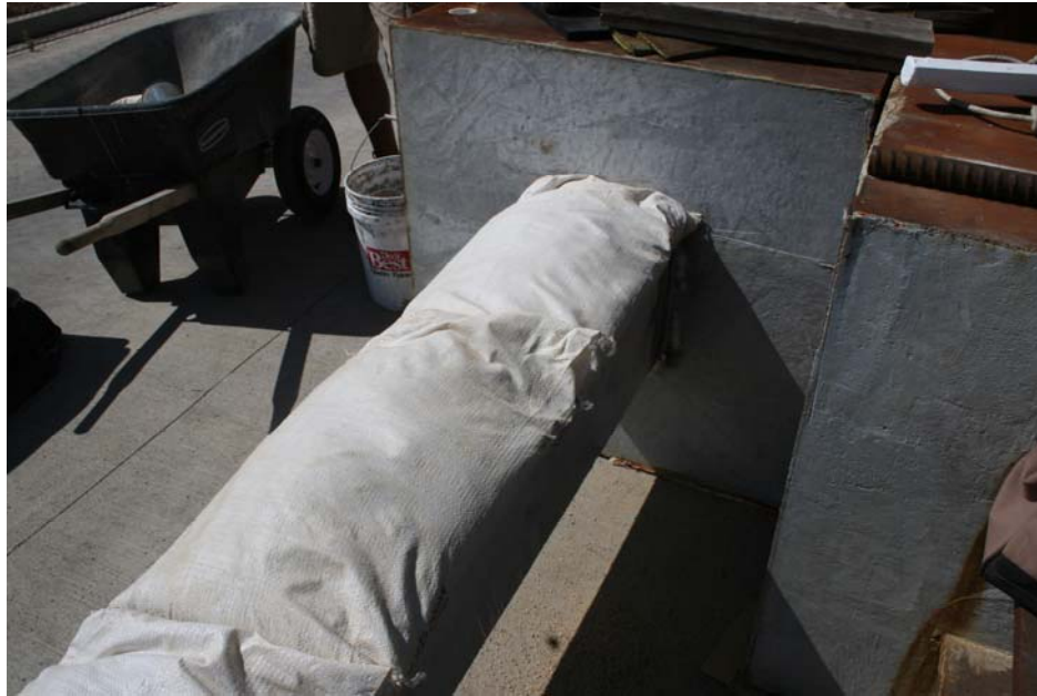
Figure 5.18: Sand Bags Laid on Top of Column
