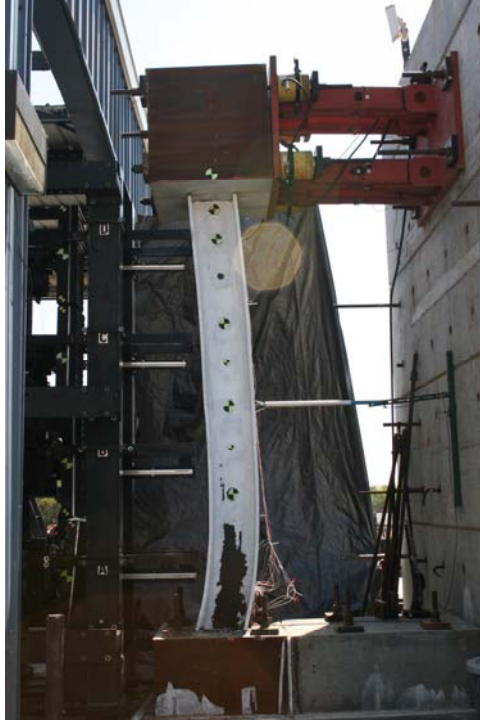
Figure 3.48: Test SA07 Column Post-Test
