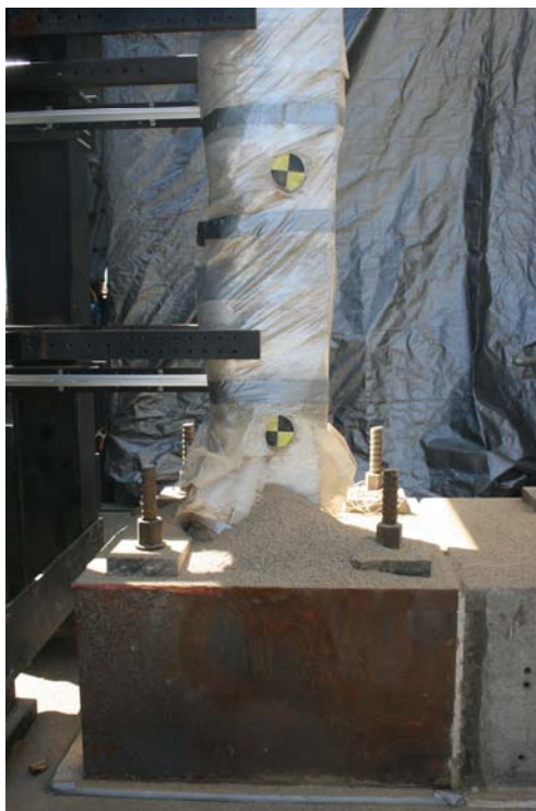
Figure 5.26: Test WA01 Column Base Post-Test
