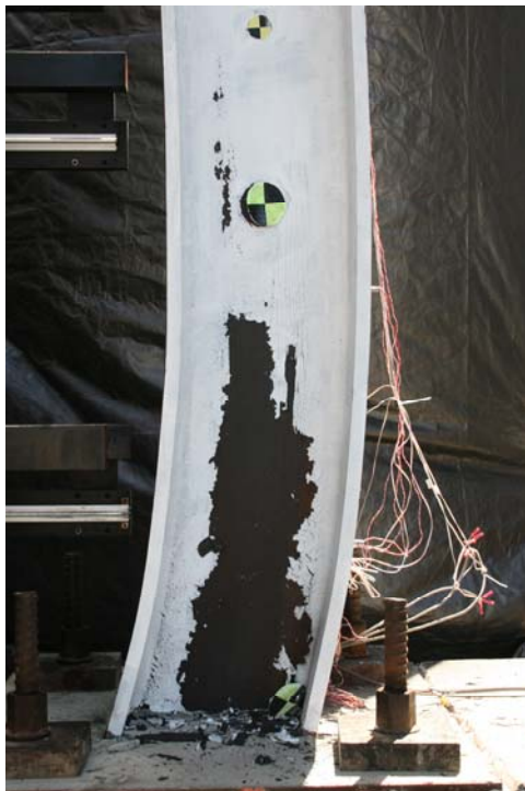
Figure 3.49: Test SA07 Column Base Post-Test
