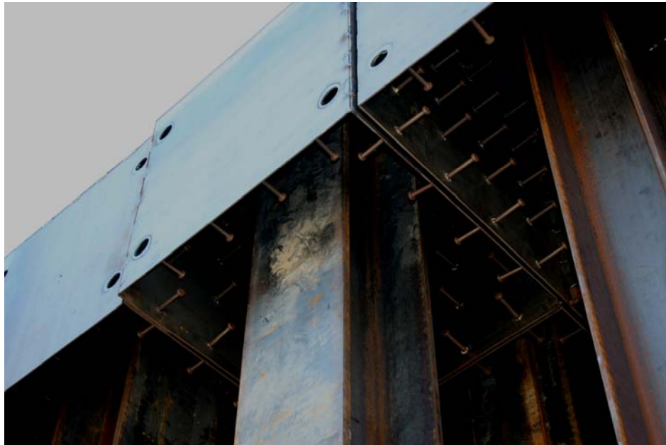
Figure 3.11: Fabricated Steel Casings with Nelson Studs
