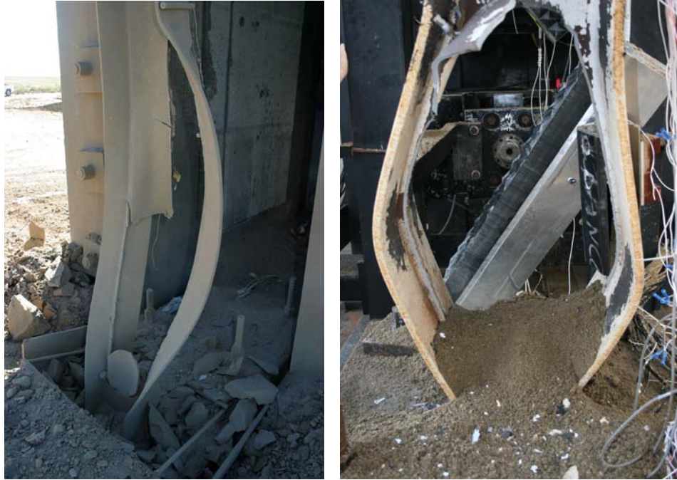
Figure 5.73: Field Test 9 (left) and WA06 (right) Column Base Comparison
