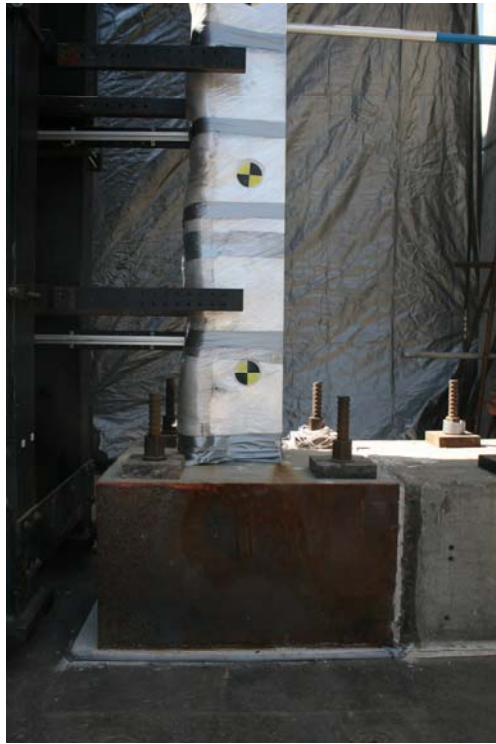
Figure 5.22: Test WA01 Column Base Pre-Test
