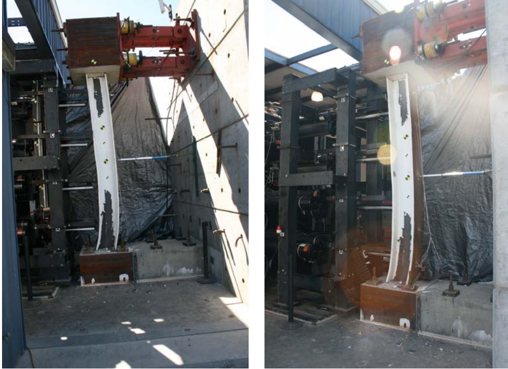
Figure 3.54: Test SA09 Column Post Test
