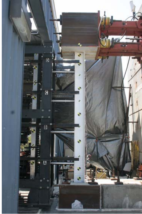
Figure 3.39: Test SA03 Column Pre-Test
