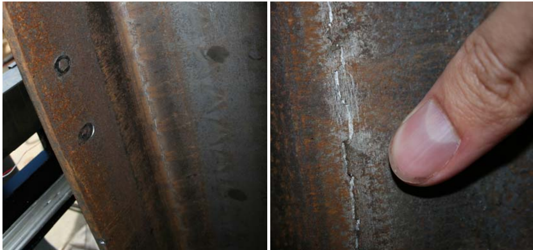
Figure 6.44: Crack Initiation from 20 m/s Test
