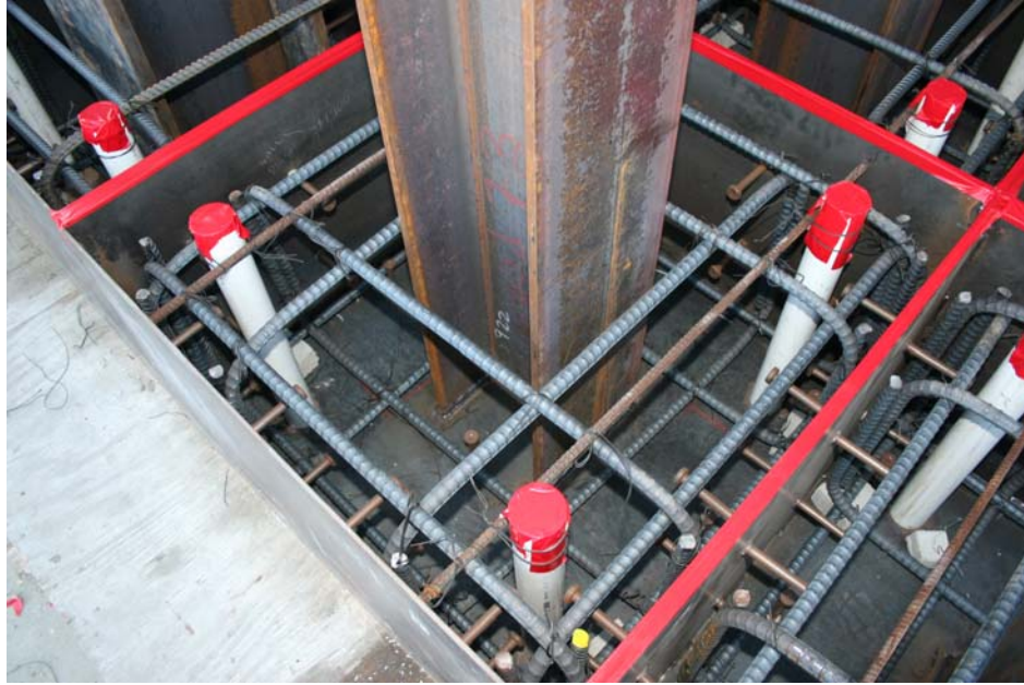
Figure 3.12: Rebar Cage in Steel Casing
