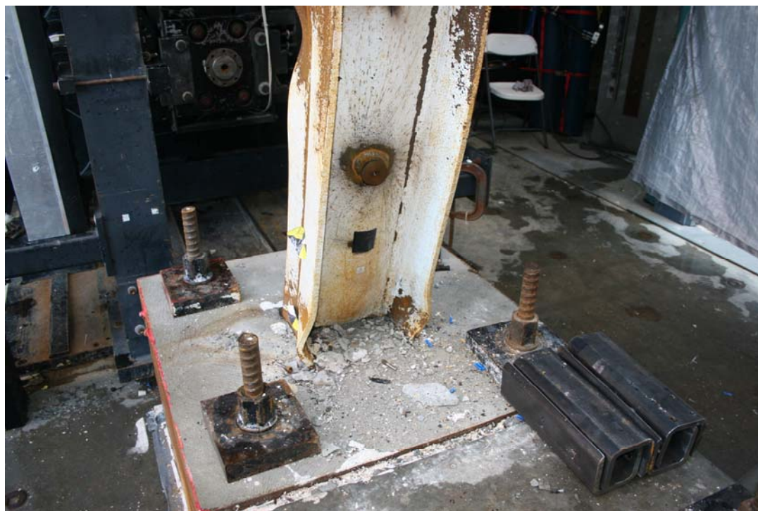
Figure 5.56: Test WA05 Base Post-Test (Non-impact side)
