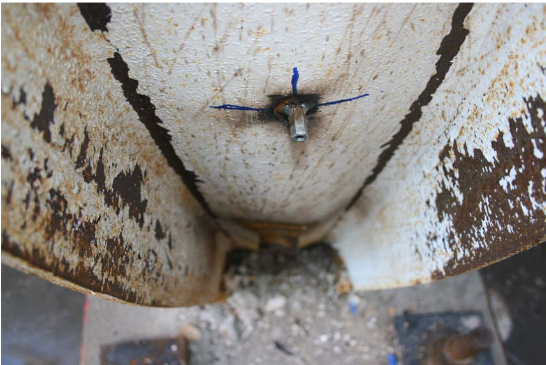
Figure 5.58: Test WA05 Column Web Post-Test
