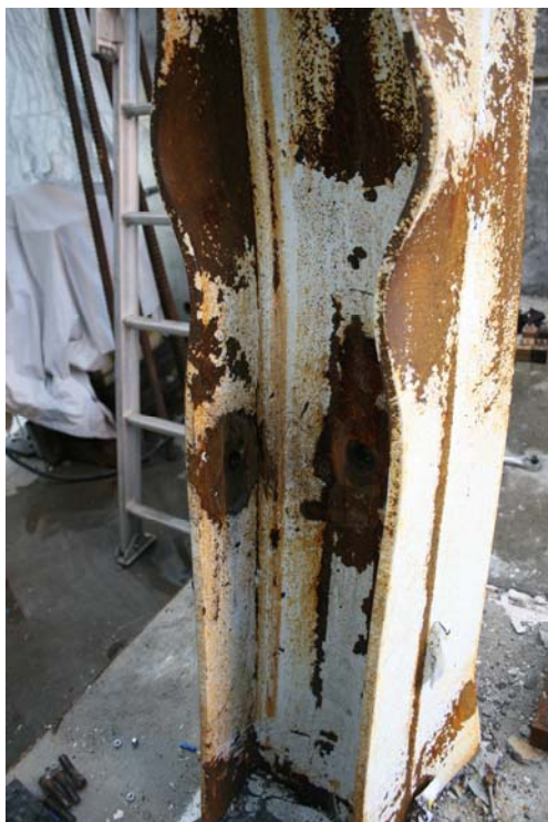
Figure 5.55: Test WA05 Base Post-Test (Impact Side)
