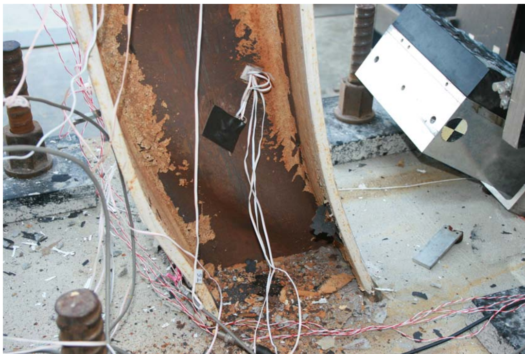
Figure 3.69: Test SA11 Column Base Post-Test (View 3)
