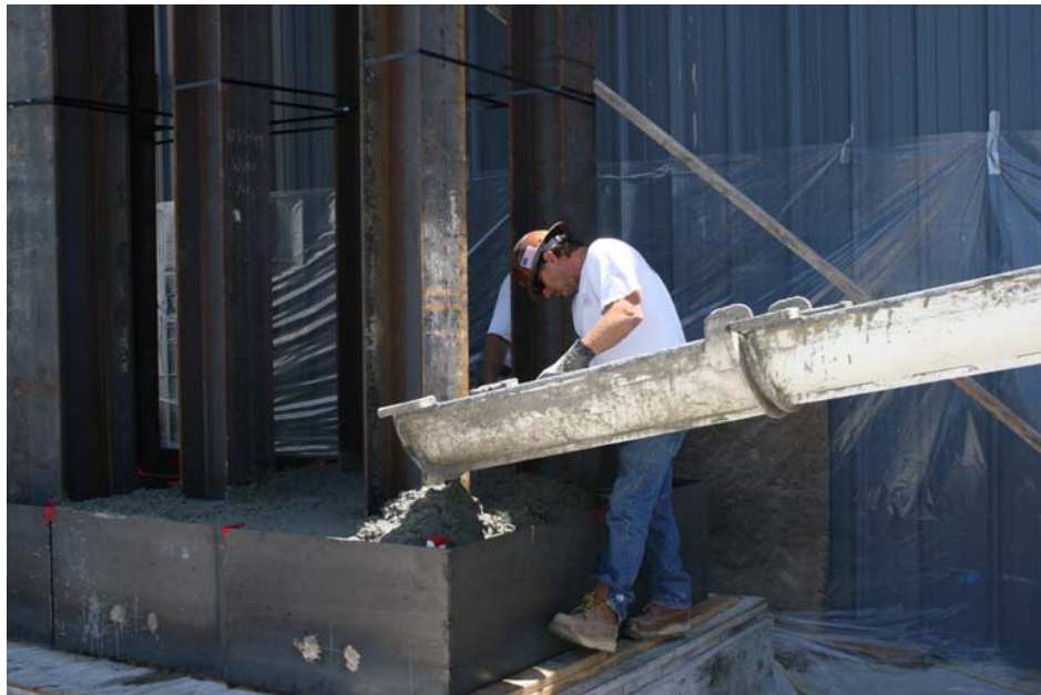
Figure 3.13: Concrete Poured into Column Base
