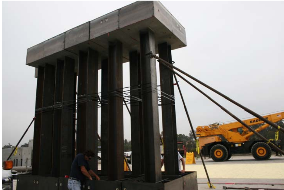
Figure 3.14: Column Specimens before Header Concrete was Poured
