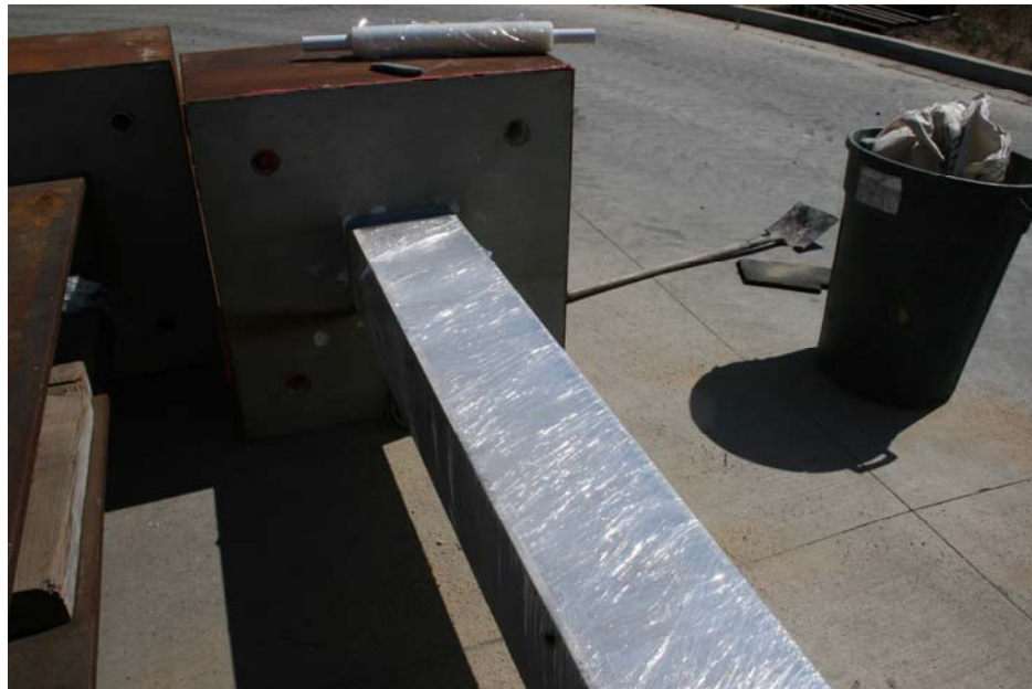
Figure 5.17: Column Wrapped with Plastic Wrap
