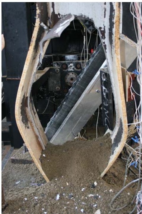
Figure 5.65: Test WA06 Column Flanges Post-Test
