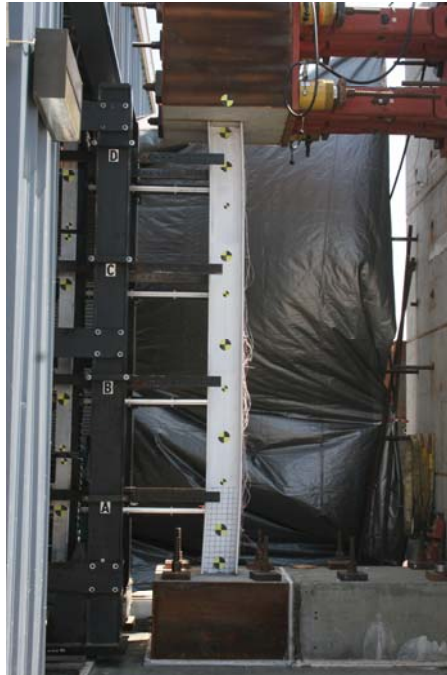
Figure 3.37: Test SA02 Column Post-Test
