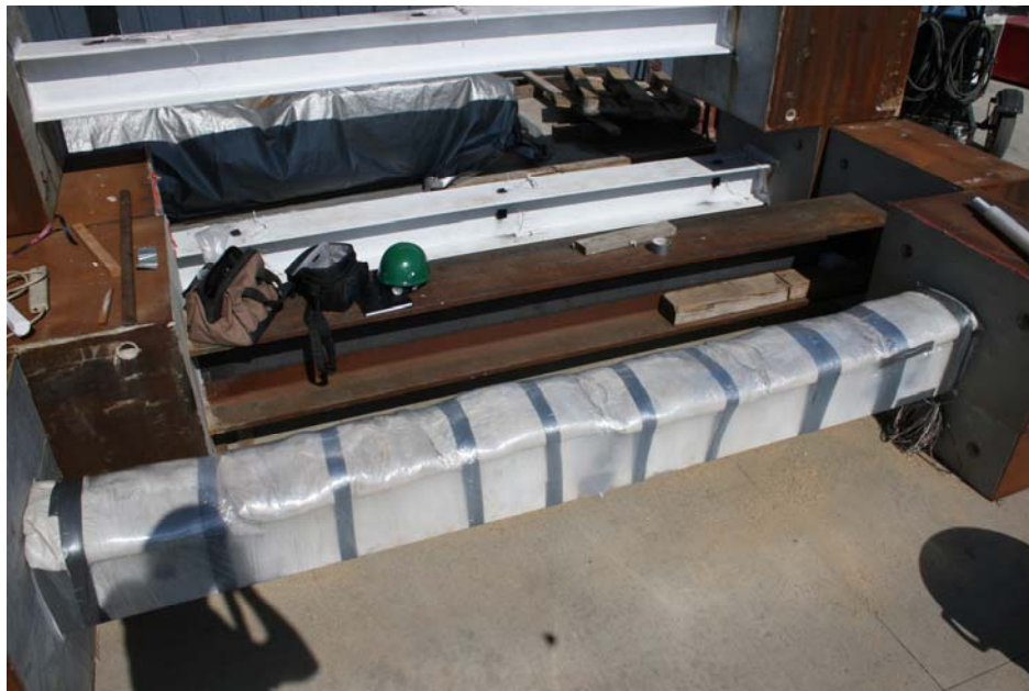
Figure 5.19: Completed Column Wrapped with Plastic and Tape
