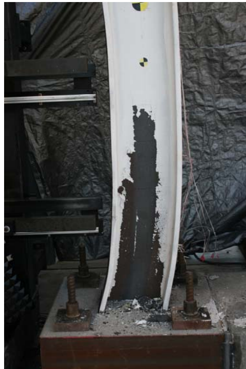
Figure 3.55: Test SA09 Column Base Post-Test
