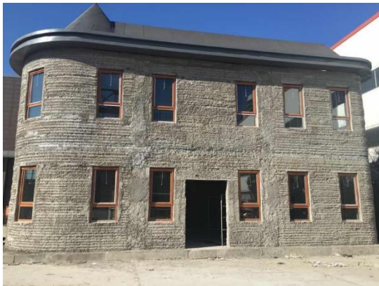
Figure 13: 3DCP ville by HuaShang Tengda [10]
