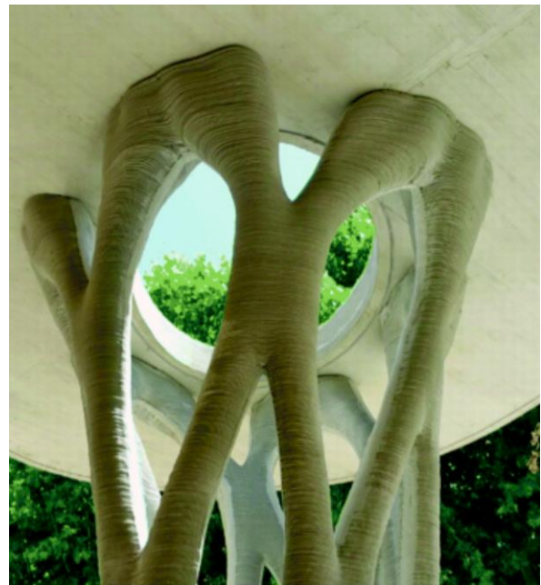
Figure 12: XtreeE pillar assembled in its final setup [14]
