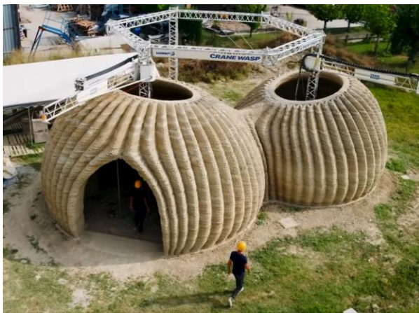
Figure 20: 3D printed dirt house by WASP [20]
