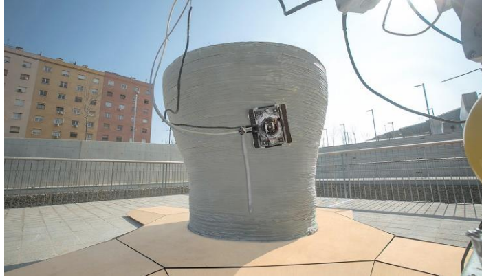
Figure 27: Vacuum minirobot reinforcing a 3D concrete printed structure by IAAC [25]
