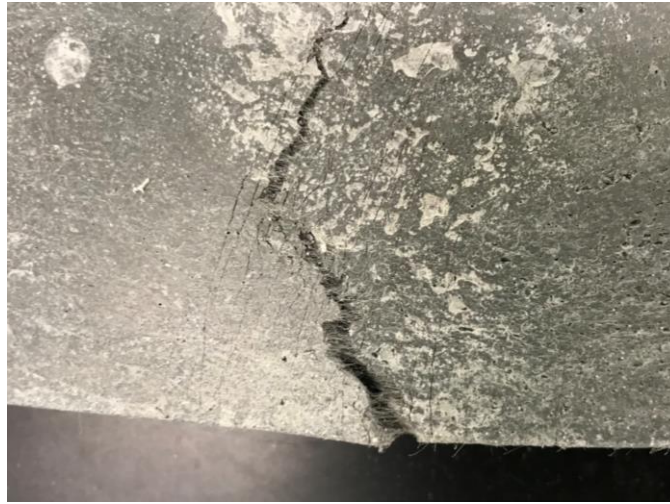
Figure 79: Close-up front view of final failure region in prismatic beam (Specimen PTV-2)
