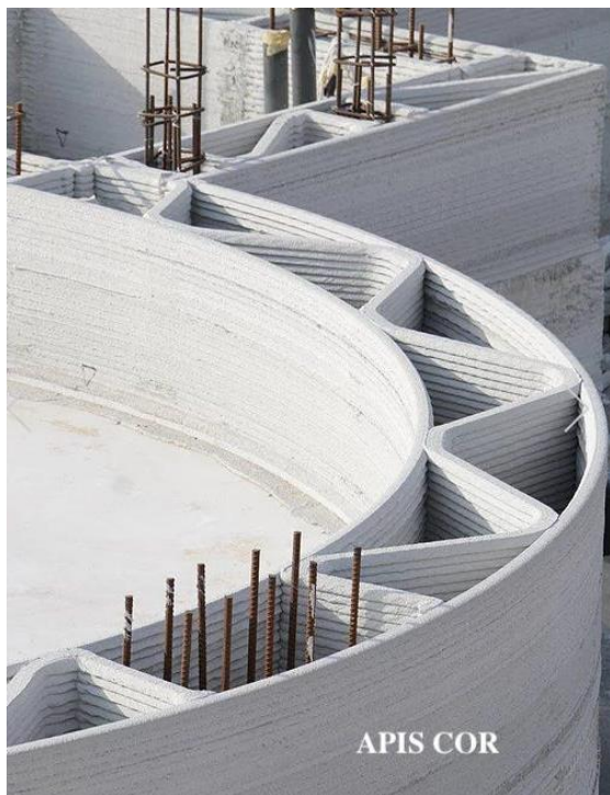
Figure 5: Steel bar reinforced 3D printed wall by Apis Cor [8]
