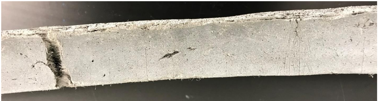
Figure 59: Damage pattern in the bottom tensile region in 3D printed topology-optimized beam (Specimen 3D-2)
