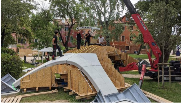
Figure 22: 3D concrete printed modular bridge being assembled [21]
