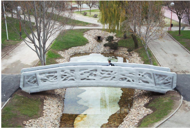
Figure 32: 3D printed pedestrian bridge using binder-jetting technique by D-shape [30]
