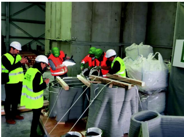
Figure 11: XtreeE pillar being transported by parts [14]
