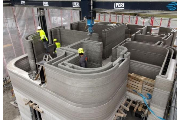
Figure 17: PERI 3D printing a house in Germany while workers install utilities [18]
