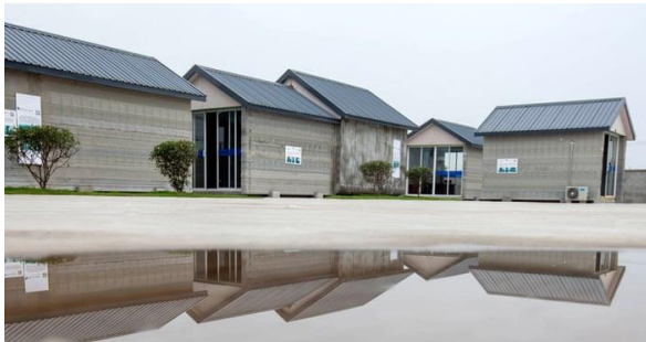
Figure 8: Winsun 3D printed 10 houses completed in 1 day [11]
