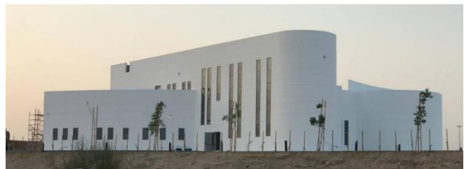
Figure 7: World's biggest 3DCP building by Apis Cor [9]
