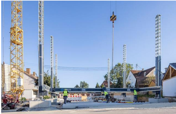
Figure 16: PERI 3D concrete printer 'OBD2' from COBOD [18]
