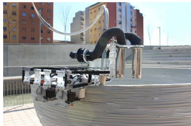
Figure 26: Grip robot 3D concrete printing a structure by IAAC [24]
