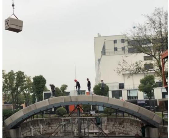
Figure 29: Modular installation of a 3DCP bridge by Tsinghua University [26]
