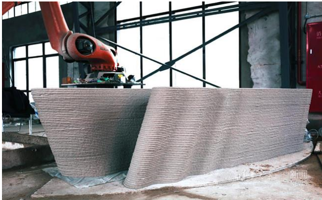
Figure 30: 3D concrete printing a modular bridge by Tsinghua University [26]
