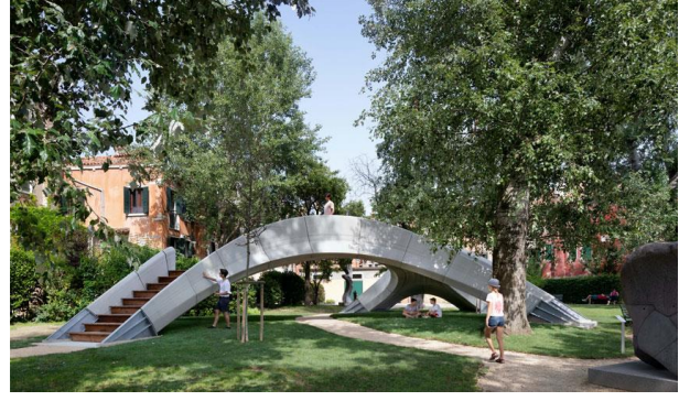
Figure 23: Completed modular 3D printed bridge by ETH Zurich [21]
