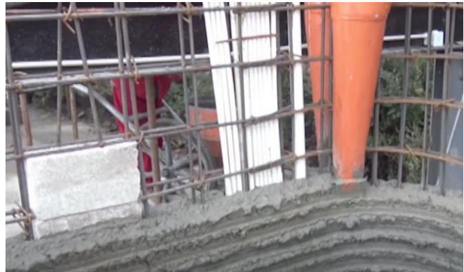
Figure 14: HuaShang Tengda 3D printing process with a forked nozzle [15]
