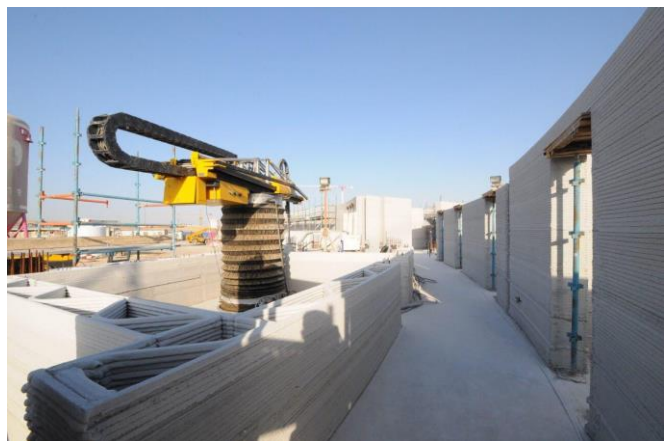
Figure 6: Apis Cor 3D concrete printing crane [8]
