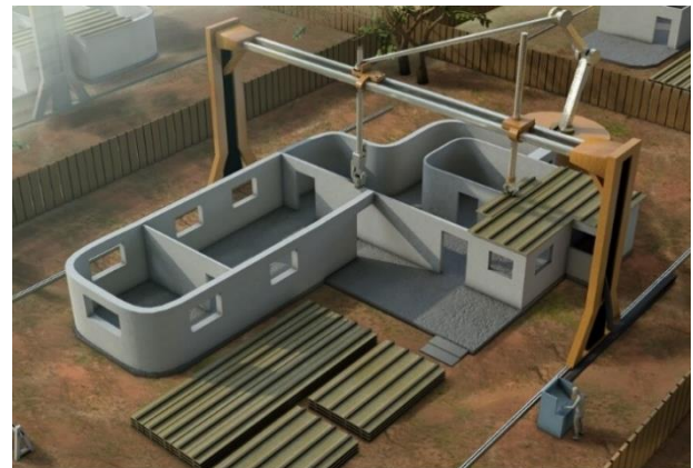
Figure 4: Contour Crafting plan to 3DCP a house [5]
