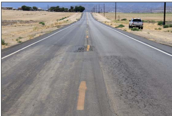
Figure 2.5: Fatigue cracking.
