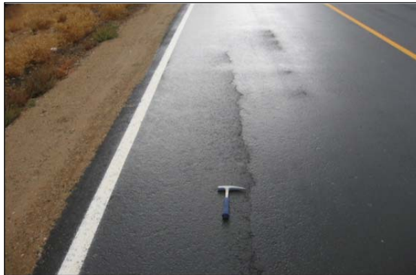
Figure 2.2: Longitudinal crack.
