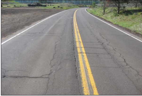
Figure 2.3: Block cracking.
