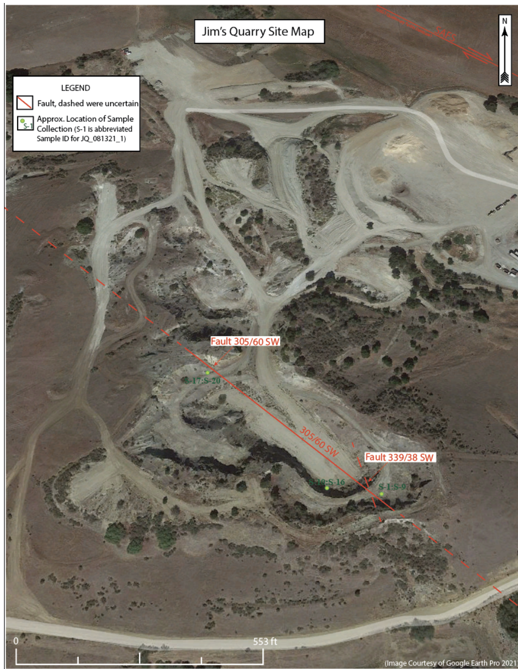
Figure 6. Jim's Quarry site location map. Red line in upper right-hand corner depicts the mapped SAF trace from the USGS Quaternary Faults database. Red lines in the quarry body are faults mapped by the author during site reconnaissance on August 13, 2021. Green dots show approximate sample location areas, with S-1, S-2, etc. as abbreviations for sample JQ_081321_1, JQ_081321_2, etc. (Satellite image from Google Earth Pro 2022).
