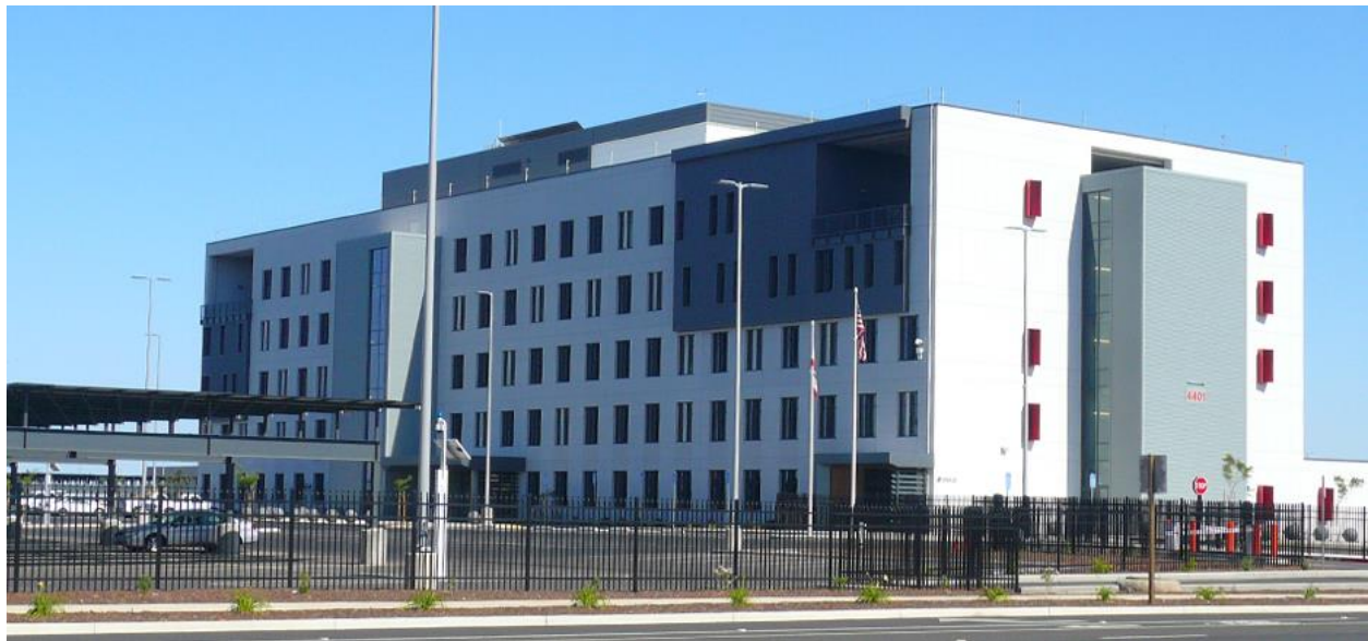
Figure 17: Photograph of SMUD East Campus Operations Center, Sacramento
