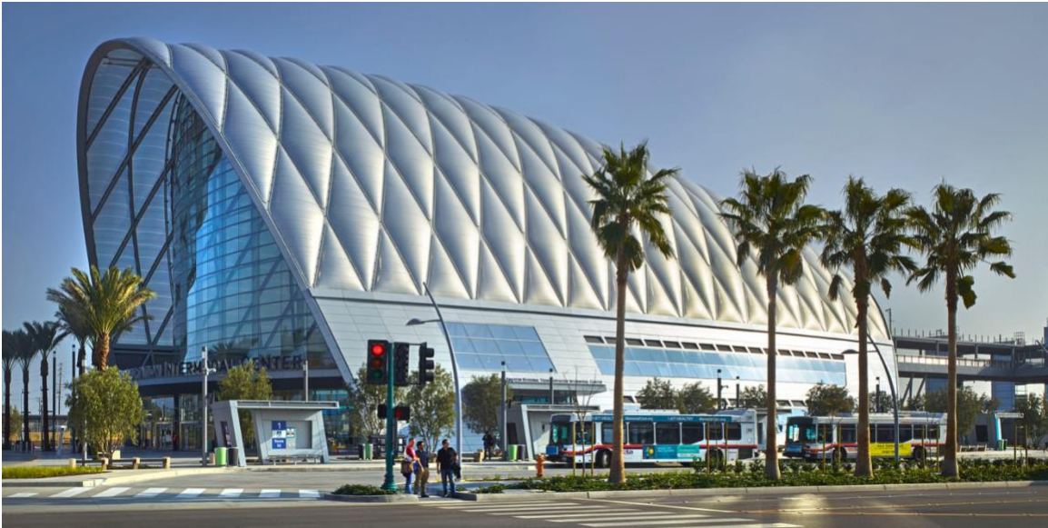
Figure 14: Anaheim Regional Transportation Intermodal Center (ARTIC)
