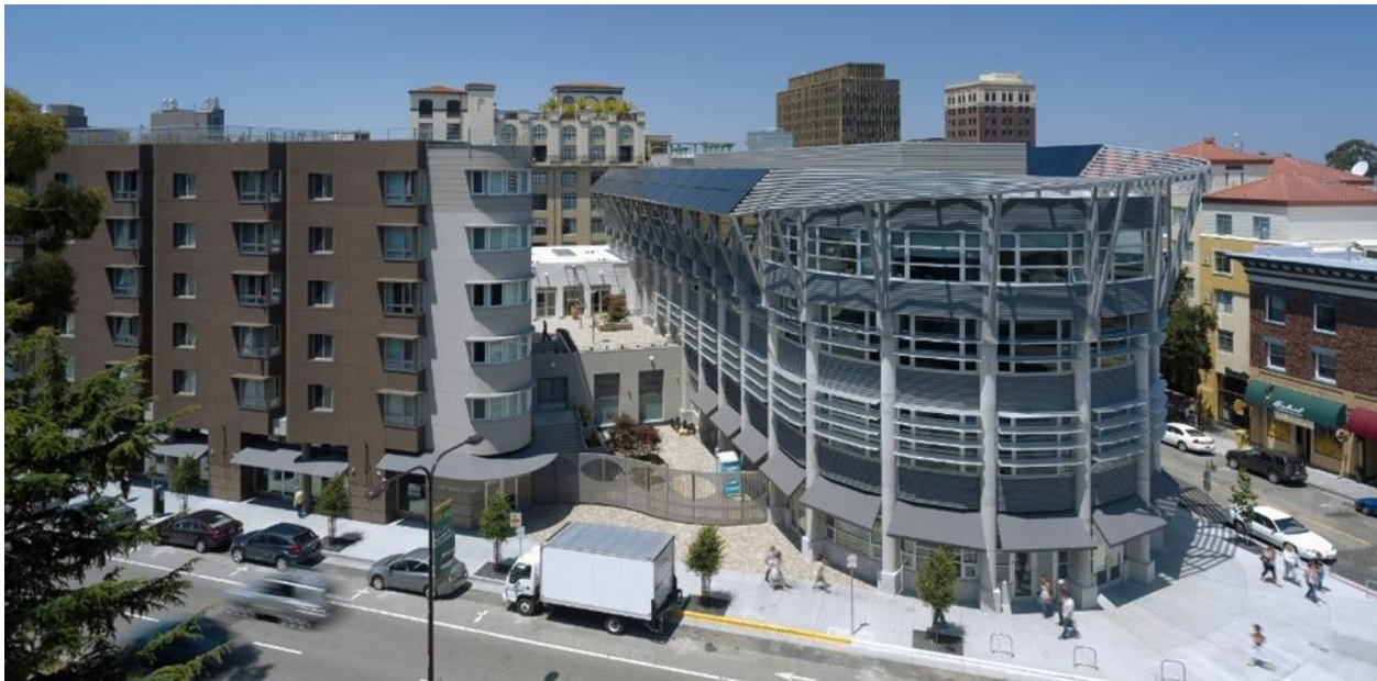
Figure 20: Photograph of David Brower Center's east and south facades
