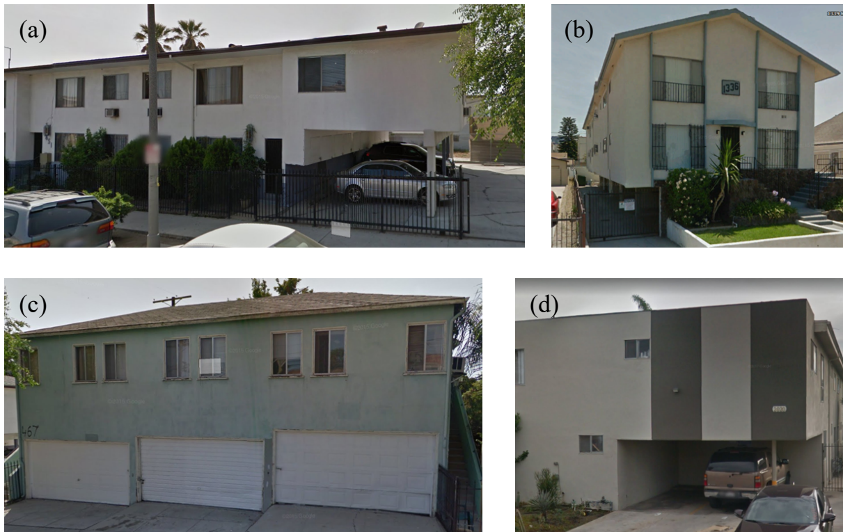
Figure 2.5 Photos of typical Los Angeles SWOF woodframe building configurations: (a) L1, (b) L2, (c) L3 and (d) L4
