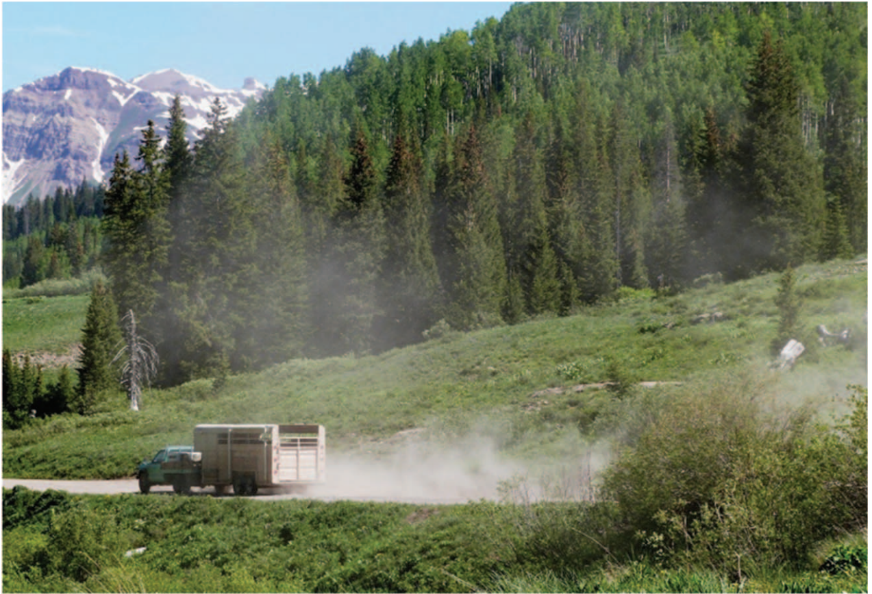
Fig. 2 A noticeable dust plume follows vehicles traveling on the unpaved roads used in this study, except during periods of rain.
