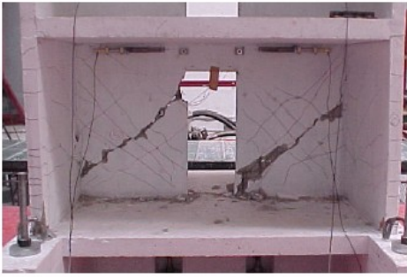
(a) Shear Failure in the First Story
