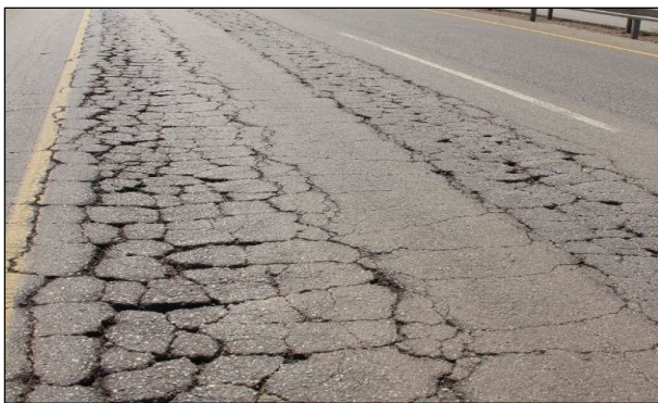
Figure 3.34: Loose blocks in severe alligator cracking.
