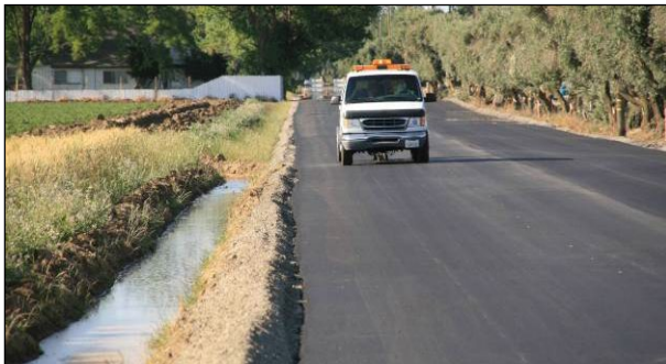
Figure 3.28: Side drain used for irrigation water.
