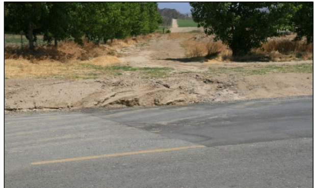
Figure 2.2: Example of road below natural ground level.
