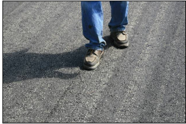
Figure 2.40: Sasobit: Shearing during final rolling.
