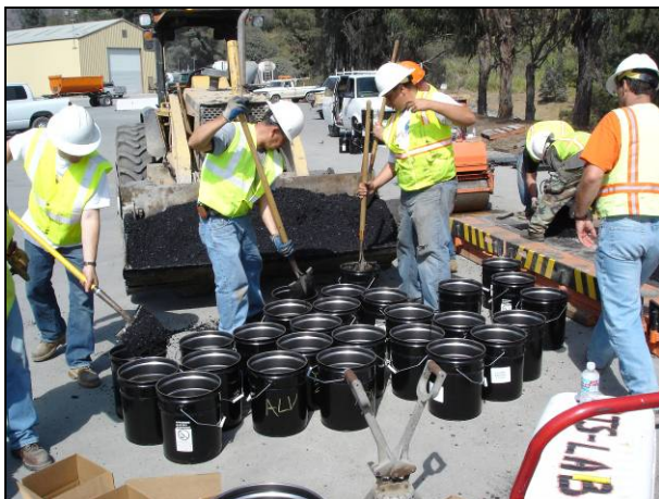
Placing loose-mix into buckets
