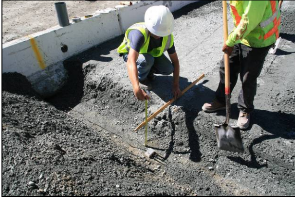
Figure 2.10: Installation of moisture sensors.
