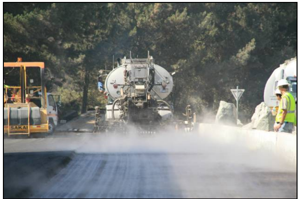
Figure 2.42: Tack coat application (Sasobit).
