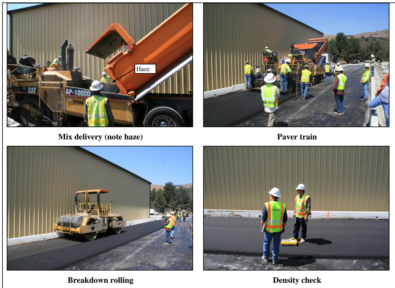
Figure 2.29: Control: Placement of first lift of asphalt concrete.
