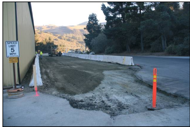
Figure 2.7: K-rail placement and subgrade/subbase preparation.
