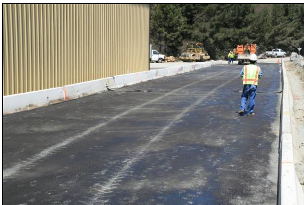
Figure 2.26: Water spray prior to priming.
