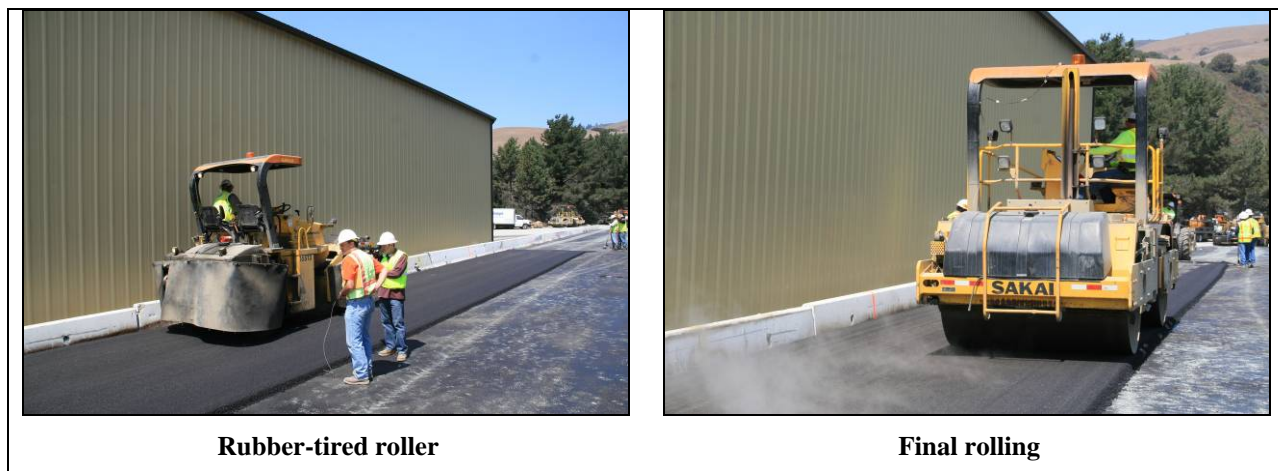
Figure 2.29: Control: Placement of first lift of asphalt concrete ( continued ).
