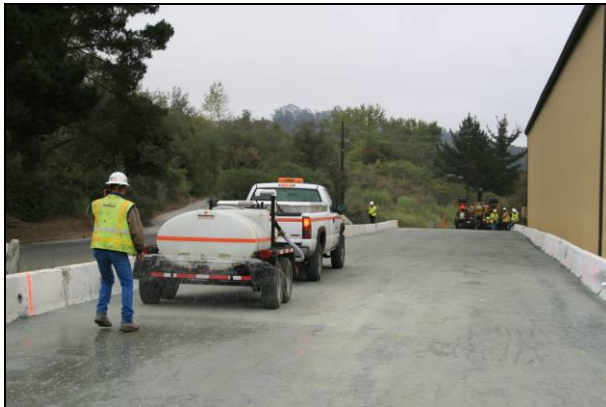
Figure 2.26: Water spray prior to priming.
