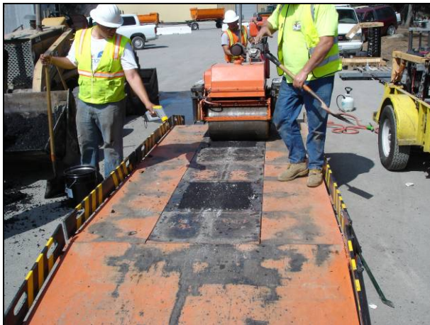
Rolling-wheel compaction/temperature control
