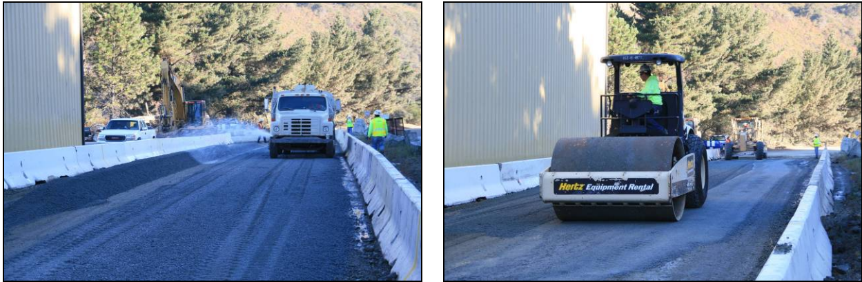
Figure 2.8: Base-course construction (continued).
