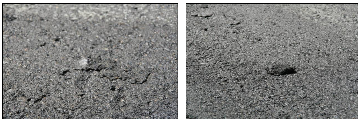
Figure 2.30: Control: Pick up during rubber-tire rolling.
