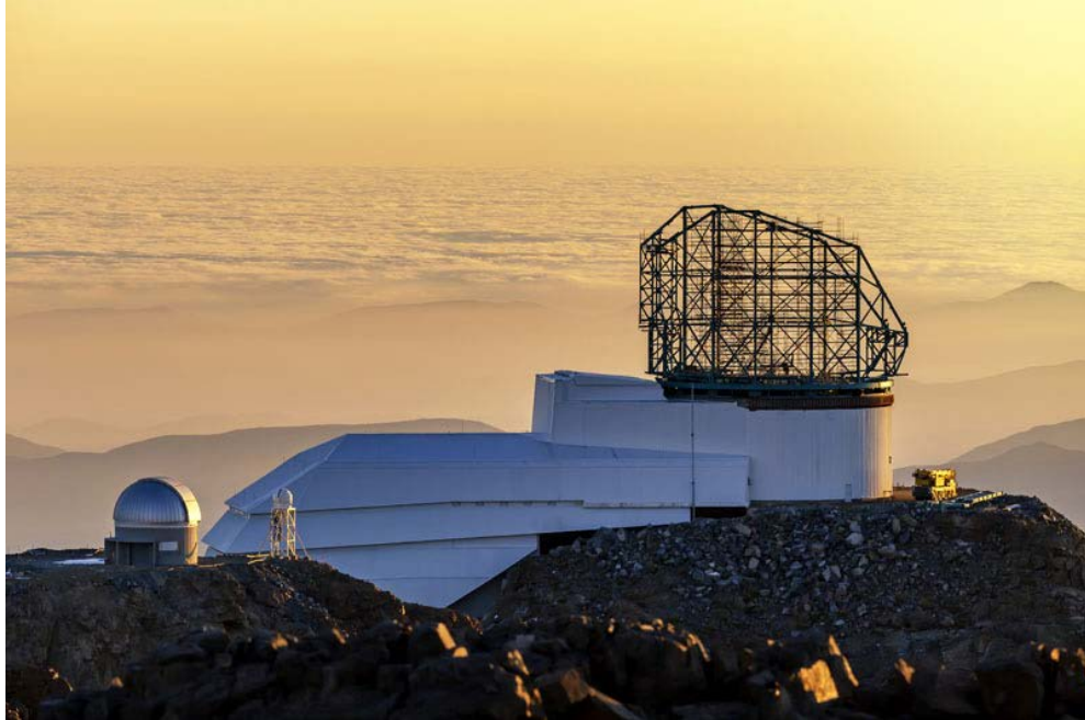
Figure 3. The Rubin Observatory in Chile, under construction in 2019.
