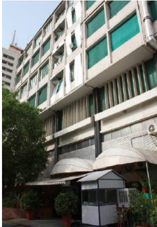
Figures: (Left) At the Paharpur Business Center (PBC), Delhi, light-colored tiles on the roof and cool wall paints were used to decrease envelope heat gain. (Right) The chart shows a drop in surface temperatures using cool materials and paints on a typical April day (Source: PBC).
