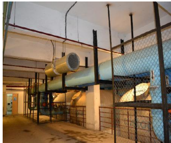
Figures: Pictures of the ethylene glycol storage system at Nirlon Knowledge Park, Mumbai.
