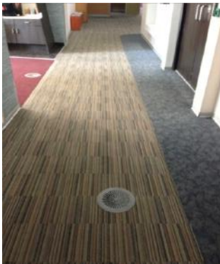
Left: picture of the underfloor air distribution outlets in the office spaces. Center: conference room with UFAD and ceiling-mounted split air system, with punched windows for diffused light. Right: the server room with a ceiling diffuser for ventilation and individual air conditioner for cooling.
