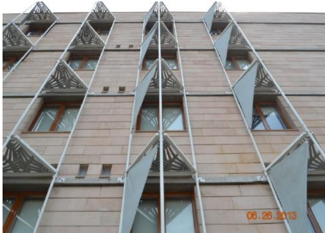
(Left): The windows at SMSF, Gurgaon, are shaded by sails that are oriented to optimally reduce solar radiation. (Right) A gentler microclimate is created using large shading devices such as garden pergolas and rooftop solar.
