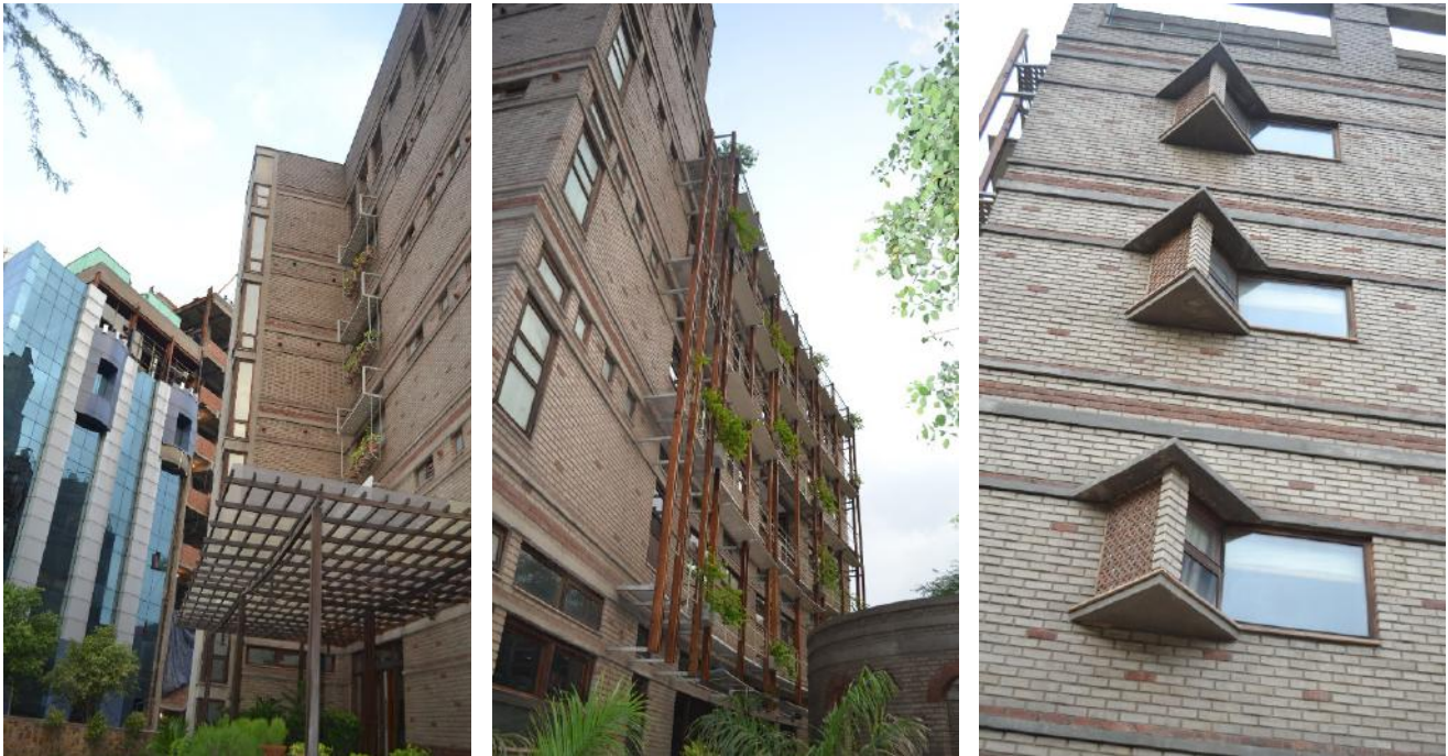
Figures: (Left) The high thermal mass of the Development Alternatives Headquarters contrasts with neighboring BAU-2 building with a curtain wall façade. (Center) The WWR was kept to a minimum, while vertical green provides visual and thermal relief. (Right) The operable windows on the western façade are innovatively angled to catch the gentler northern and southern solar exposures.
