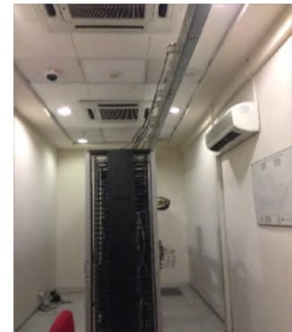
Left: picture of the underfloor air distribution outlets in the office spaces. Center: conference room with UFAD and ceiling-mounted split air system, with punched windows for diffused light. Right: the server room with a ceiling diffuser for ventilation and individual air conditioner for cooling.
