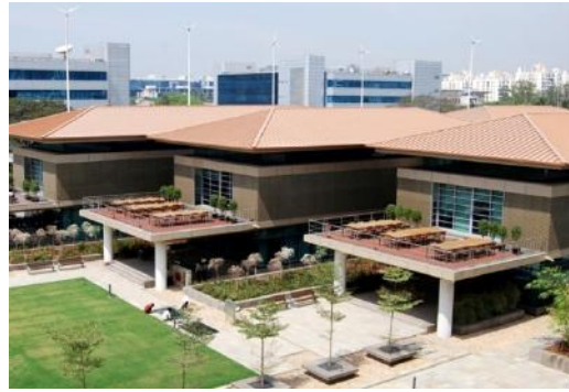
Figures: Naturally ventilated spaces at SDB-1 on Infosys Pocharam campus, and at Suzlon One Earth campus. (Left) The cafeteria at Infosys, Pocharam, utilizes natural ventilation enhanced with breezeway and ceiling fans in dining and interaction spaces despite high occupancy density. (Right) Small terraces interspersed between office blocks serve as attractive break room spaces at Suzlon One Earth in Pune (photo: Synefra).
