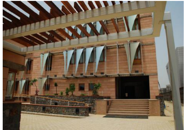
(Left): The windows at SMSF, Gurgaon, are shaded by sails that are oriented to optimally reduce solar radiation. (Right) A gentler microclimate is created using large shading devices such as garden pergolas and rooftop solar.
