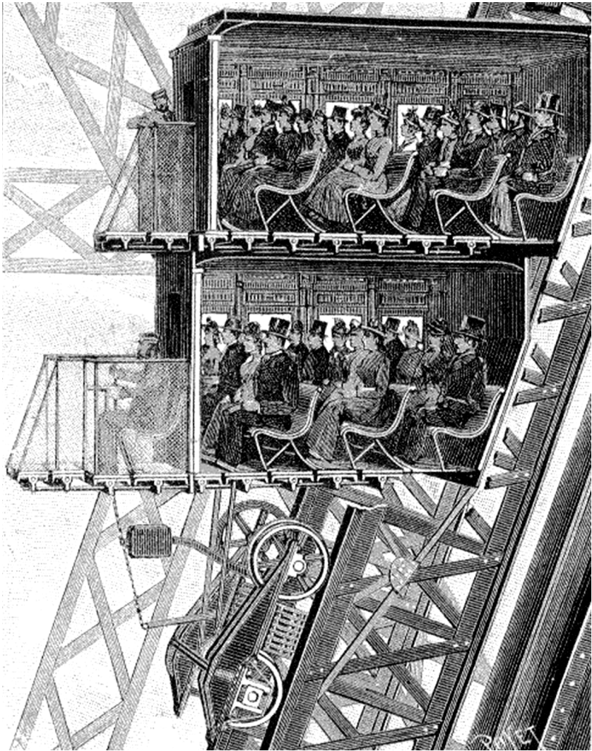
Figure 4: Cross section view of Otis Elevator on the Eiffel Tower, La Nature , May 4, 1889, volume 17, p. 360
