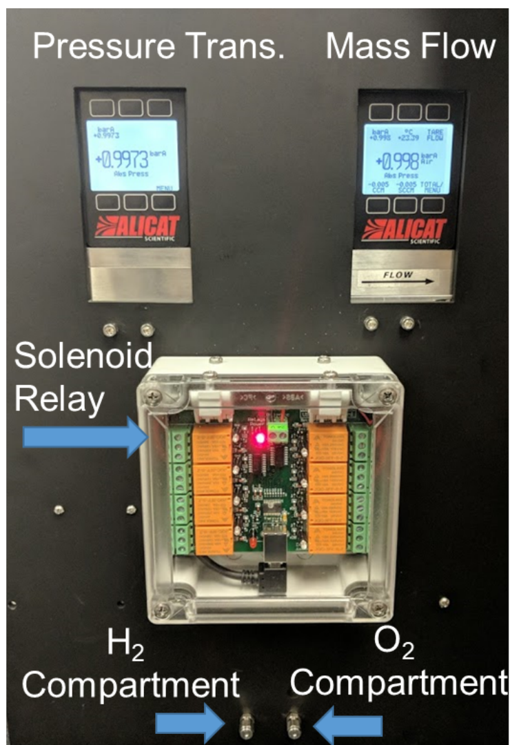
Figure 3. 11 Front of completed panel.
