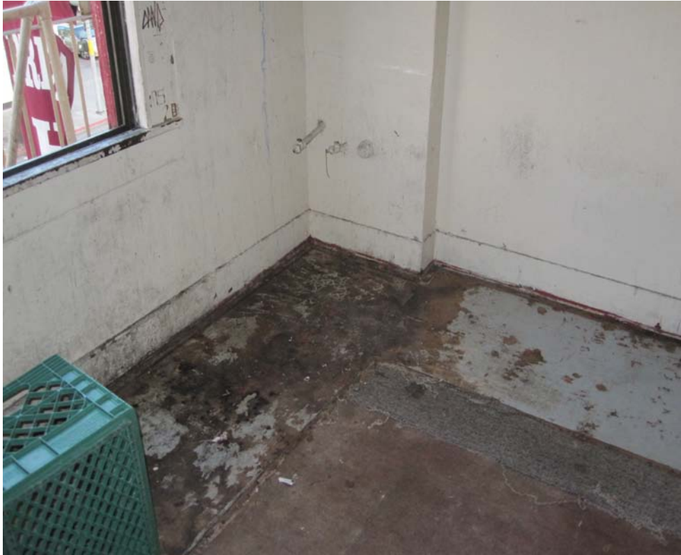
Floor stained and eaten away from a bedbug infestation. The carpet has been pulled up. Raman Hotel, October, 2009.
