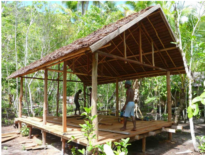
Figure 45 Beteo men construct a new homestay, Kri Island, 2012
