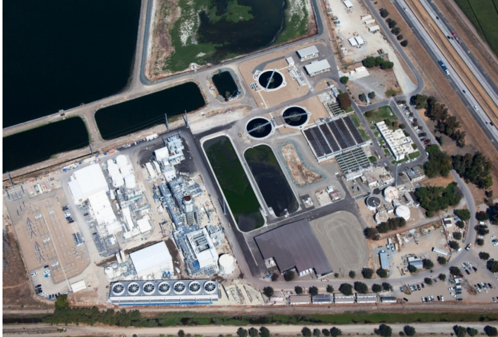
Figure 3.3 Aerial view of the Lodi Energy Center and the Lodi White Slough Facilities. (Photo courtesy of NCPA)
