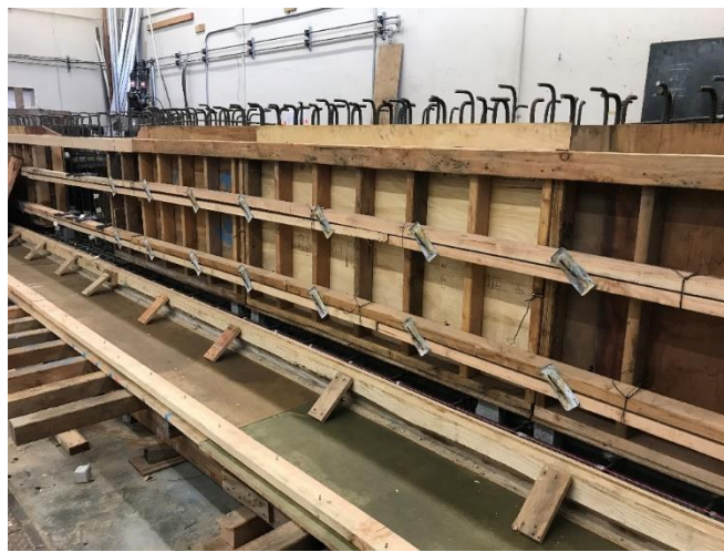
Figure 2.18: Formwork construction for specimen #2
