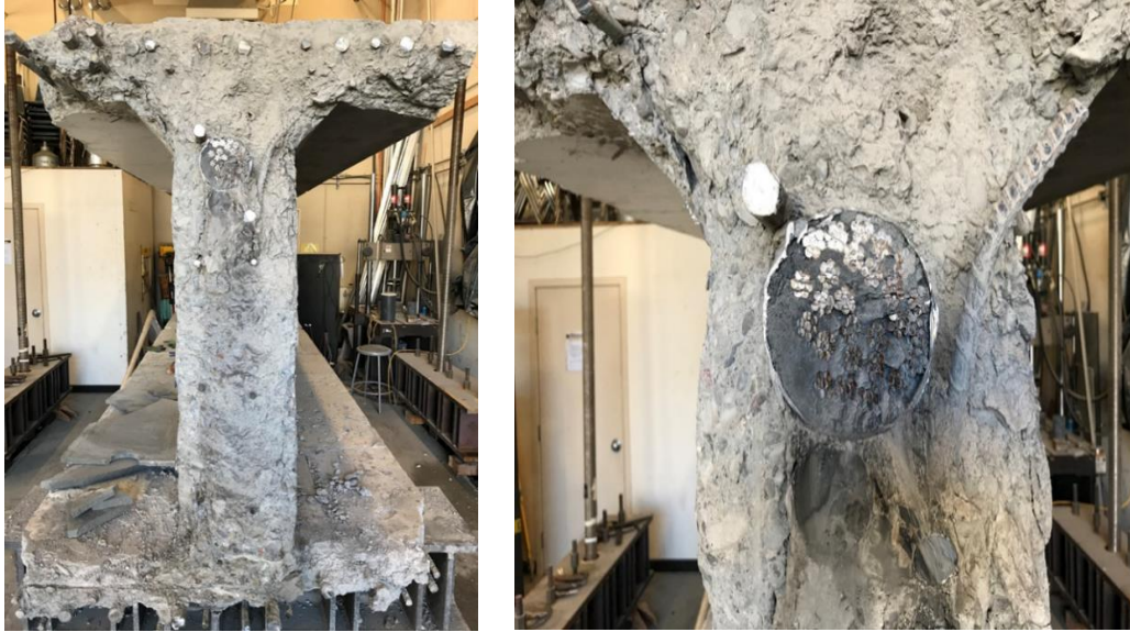
Figure 3.3: View of girder cross-section showing state of duct after testing
