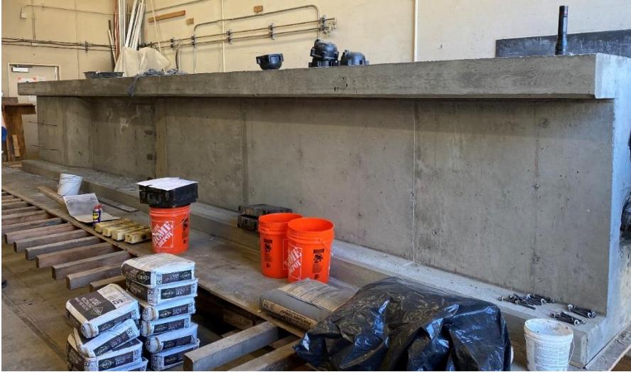
Figure 2.21: Specimen #2 after stripping formwork and ready for post-tensioning
