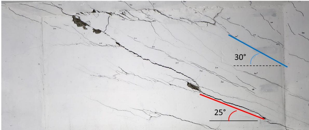
Figure 3.15: Observed inclination of diagonal cracks (specimen #2)
