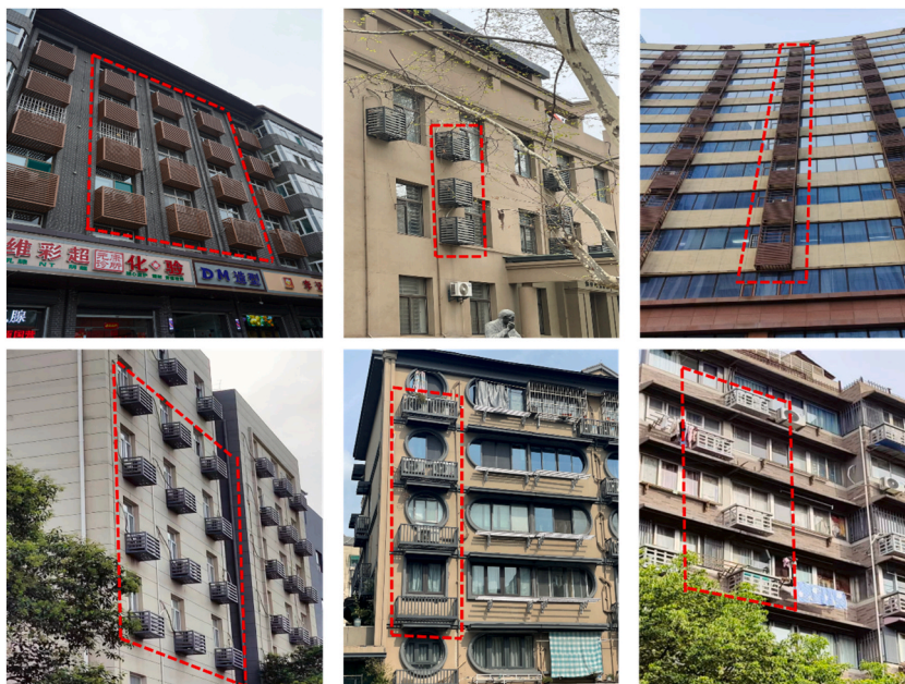
Fig. 1. Photos of the typical covers on the outdoor units of AC in some Chinese cities.
