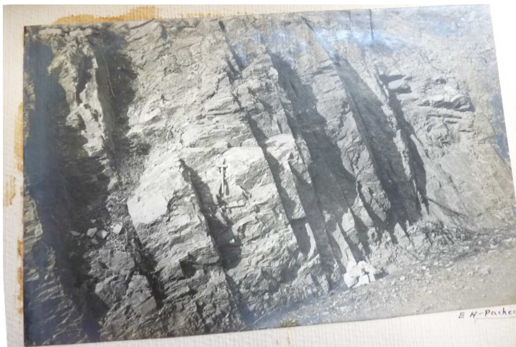
Image 1.5: “Detail of the quartz bands on the right side of the Portillo de Cíjara on which the dam will support itself. The hermetic union of the bands indicates the impermeability of the setting and the strength of bands, their excellent conditions of resistance.” 90 Eduardo Hernández-Pacheco and Gumarsindo Gutiérrez Gándara, “Informe relativo a las condiciones, ACHG.”
