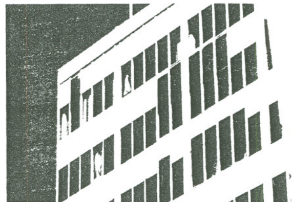
Figure 6-34. Detail of south elevation.
