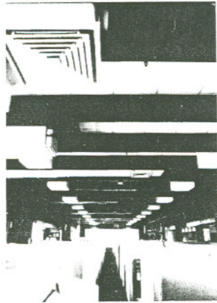
Figure 6-47. Typical office ceiling.
