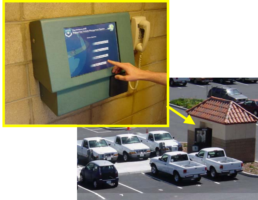
Figure 1. Touchscreen kiosk terminal (located inside small building) used to check-out shared-use vehicles (electric pickups and electric city cars).
