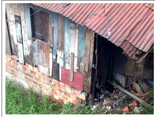
Figure 15. Photo of a house in Tabatinga, Brazil, clad with a combination of industrial materials including the predominant calamina (galvanized steel). © Maria Paz Gutierrez.
