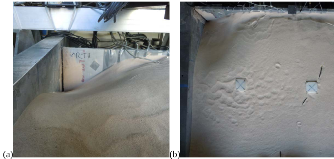
Figure 3.13: Cave in at northeast corner of structure
