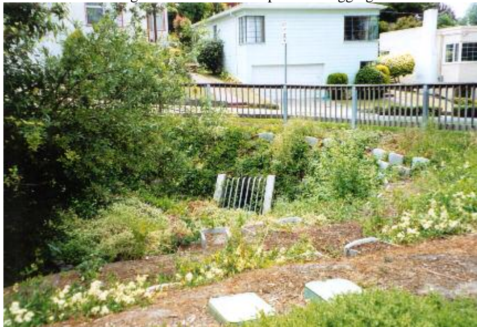
Figure 4. Photo of downstream inlet of Baxter Creek in Poinsett Park. Notice small retention basin constructed and grate over the inlet to prevent clogging from trash and debris.
