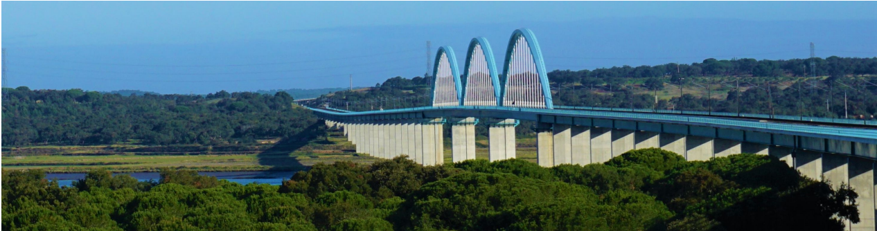
Figure 1. Overview of the Sado Bridge.
