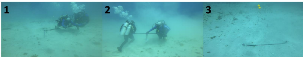
Figure S2.19 Attachment of the Arks to their mooring system. The positively buoyant Ark structures is pulled to depth using a block and tackle in order to attach the downline to the mooring system. In Step 1, the block and tackle is unspooled in order to attach one side (the end with the becket and cam) to the anchor point, and the other end to the base of the Ark mooring bridle. A safety “loop-tagline” that is attached to the Ark base and a single anchor point may be used for security in case of block and tackle failure. In Step 2, the block and tackle is engaged to pull the structure to depth. The structure is 300 lbs. positively buoyant and the block and tackle has a 6:1 purchase; thus, the force required to pull the Ark to depth is approximately 50 lbs. At the end of Step 2, the shackle at the base of the downline should be fastened to the galvanized pear-shaped link at the top of the anchor bridle, then the tension can be transferred to the mooring system and the strain gauge removed. Note: Divers should maintain continuous observation of the sand anchors to make sure they are not failing under the various loading scenarios of the installation.
