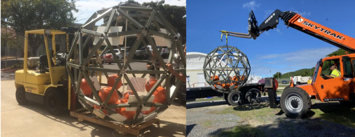
Figure S2.21 Shell Arks may be attached to a pallet and lifted via a forklift to load them onto vessels or transport them as needed.
