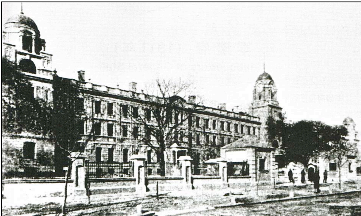
Figure 1. Supreme Court, 72 Ministry of Justice Street, Beijing, 1914. Source : “Architecture in the Chinese Capital” (1914, 356).
