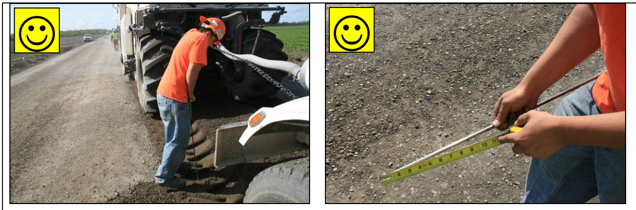
Figure 7.5: Checking mixing depth.
