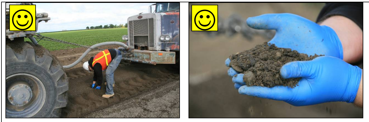
Figure 7.6: Checking material consistency and color.
