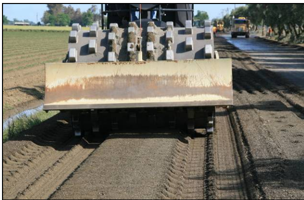
Figure 7.9: First padfoot roller pass.
