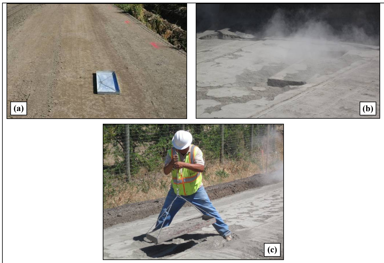
Figure 7.4: Monitoring stabilizer application rate.
