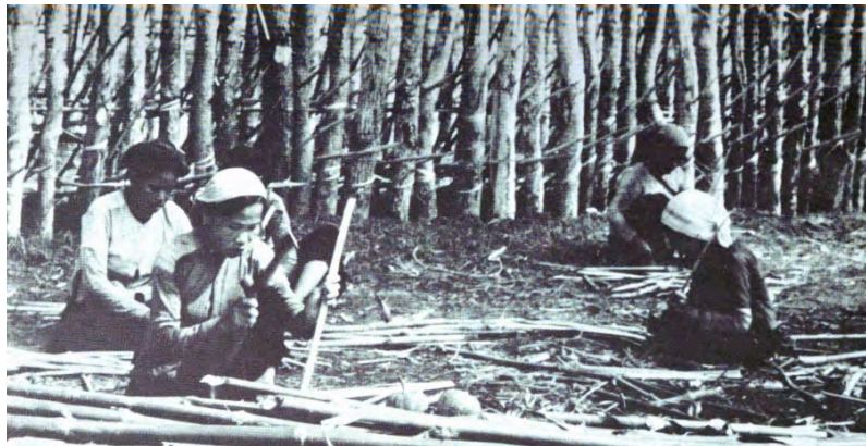
Sharpening prongs for the hamlet fence
