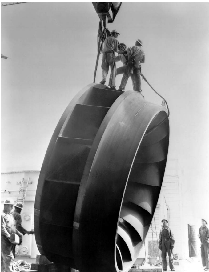
Fig 2.06 Installation of inlet scroll and Francis turbine runner at Grand Coulee Dam, September 1941. U.S. Bureau of Reclamation.
