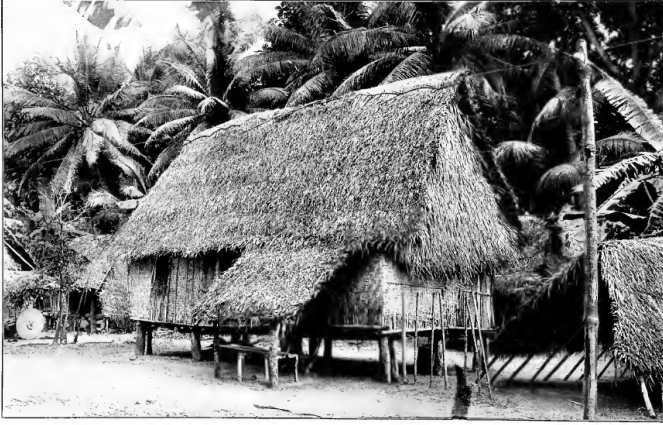
TYPICAL NATIVE DWELLING, ISLAND OF GUAM. SIDES OF BAMBOO AND WOVEN REEDS AND ROOF OF COCONUT THATCH.
