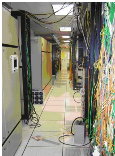
Figure 2 CRAH units in the data center
