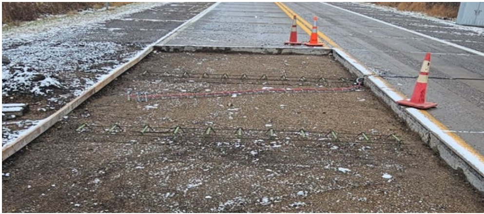
Figure 3 – Highway pavement placement under freezing conditions using a volumetric truck.
