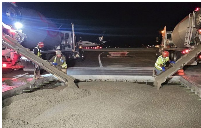
Figure 2 – Ready-mix concrete delivery on SEATAC slab replacement project.
