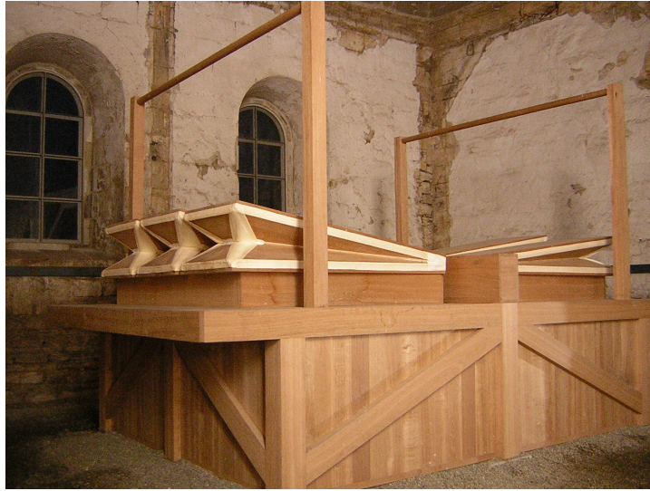
Figure 2.9. The “bellows” constructed for the Halberstadt performance of Cage’s Organ 2 .
