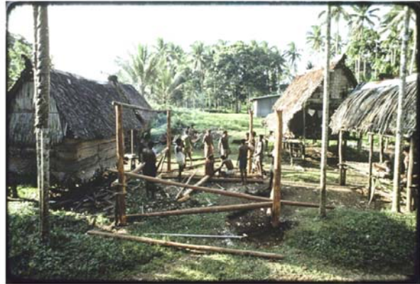
House-building: men construct frame, vertical poles are notched at top, betel nut palm (l) taboo with coconut frond tied around it, 1975. Edwin Hutchins and Dona Hutchins Collection, UC San Diego Library.
