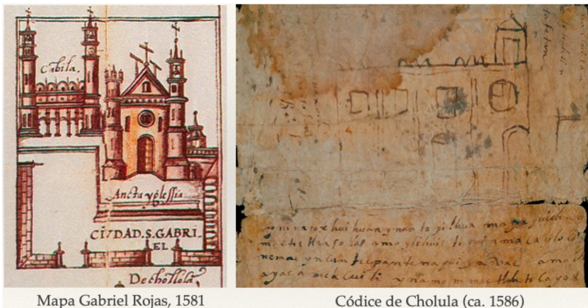
Figure 8. Historical documents from the 16th century showing the convent temple of San Gabriel Cholula with the presence of the oculus or rose window on its facade.
