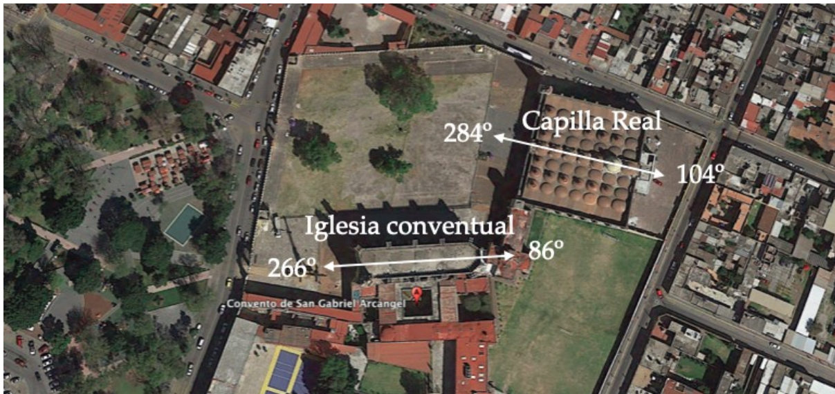
Figure 3. The convent church of San Gabriel Cholula and the Royal Chapel have a different orientation from each other (measurements indicated with the white arrows), but also different from the orientation of the city layout.
