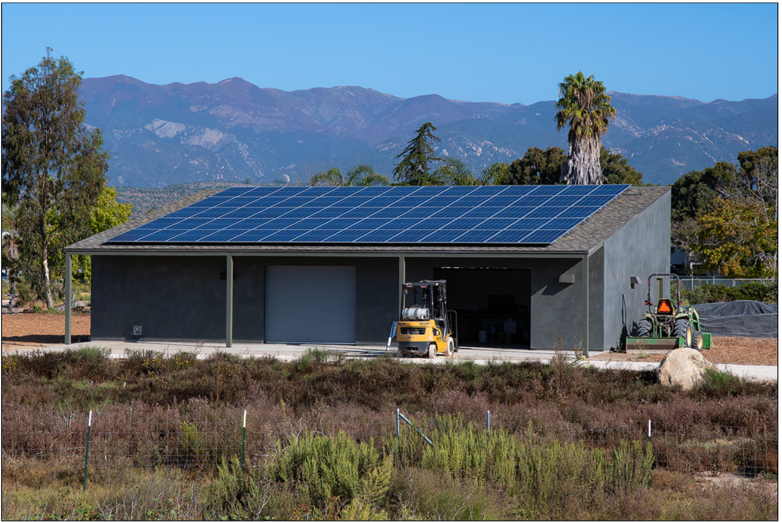
Solar panel array on the ROOST.
