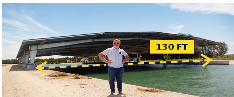
Figure 2: A picture of a solar installation above a canal in CA with a reporter for perspective.
