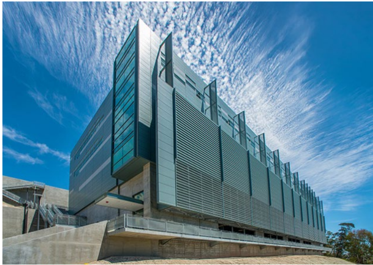
Figure 7 Building 59 at LBNL, Berkeley, California
