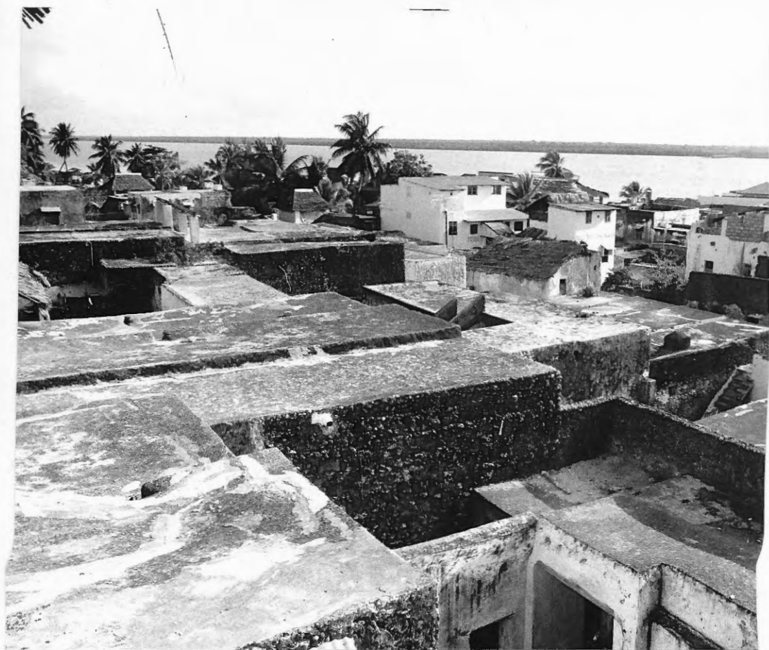
Fig. 28 Roof-top view of Lamu.
