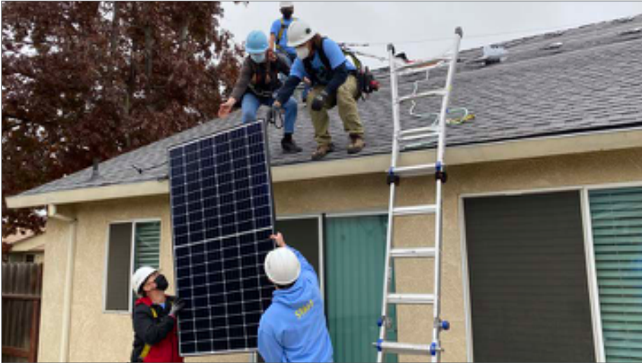
Installation of solar PV panels on a single family home in the TCC project area. Photo credit: GRID Alternatives
