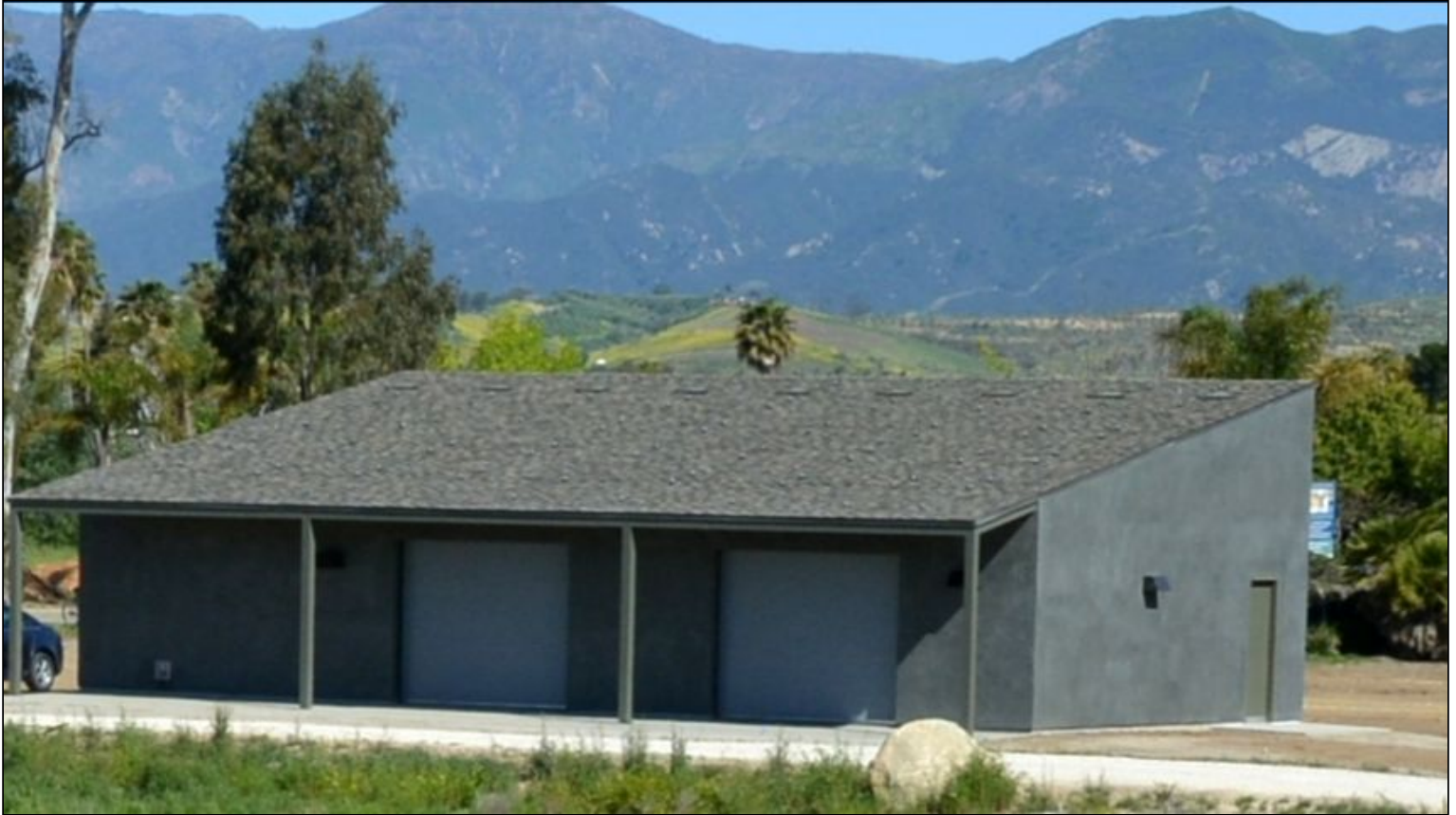
The roof of the ROOST building at NCOS will soon be covered with solar panels.
