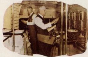
With an interior patterned after that of a standard railway mail car, the first U. S. Post Office of the Highways provides every facility for sorting and handling all classes of mail enroute.
