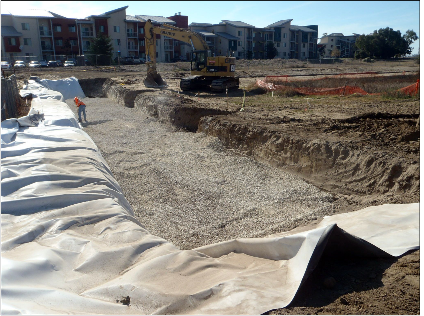
Installation of bridge supports at Phelps Creek (two top photos), and Arizona Crossing by the Sierra Madre apartments.
