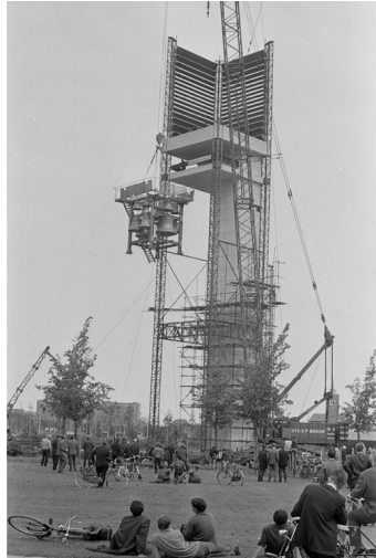
Figure 6. Locals watch as the bells of the Philips Carillon are lifted by crane into the belfry.
