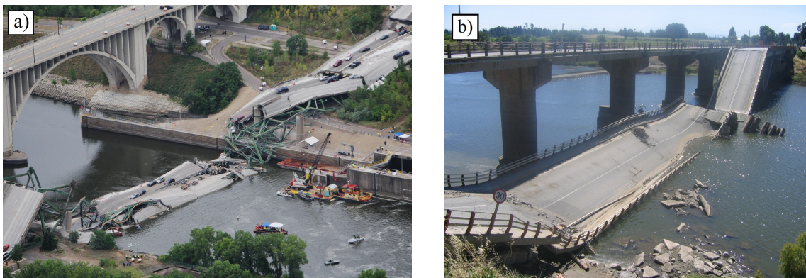
Figure 1.1: (a) Collapse of the I-35W Mississippi River bridge in Minnesota, USA, in 2007, (b) Collapse of the Loncomilla bridge in Chile in 2004.
